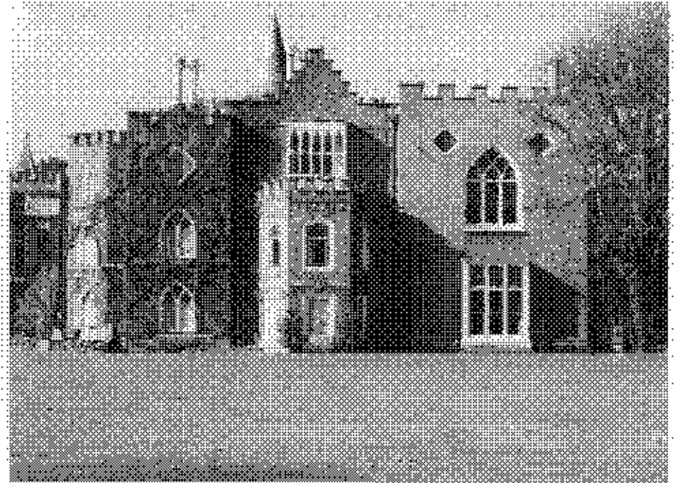
South and East Fronts
