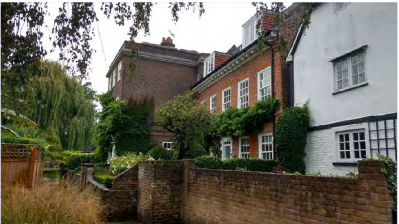
Plate 16: View towards Site from The Embankment from north-east
