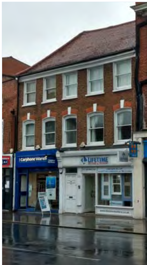
Plate 20: 10-12 King Street (Site 3) from south
