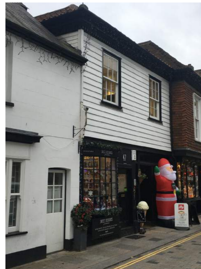
3. Weatherboard - Church Street
