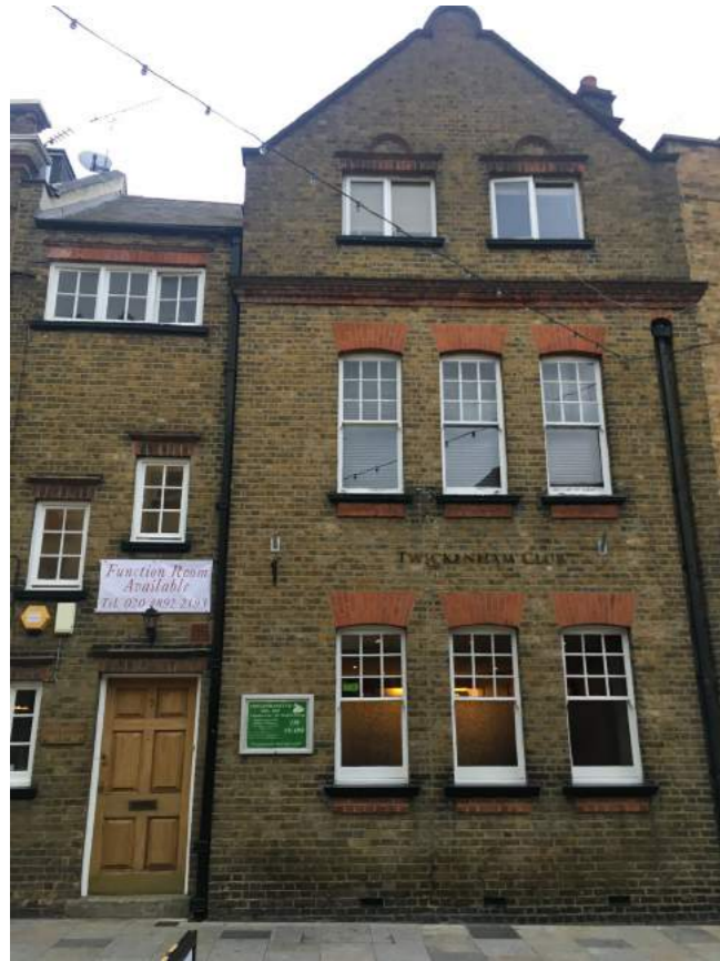
1. Brickwork Gables - Church Street
