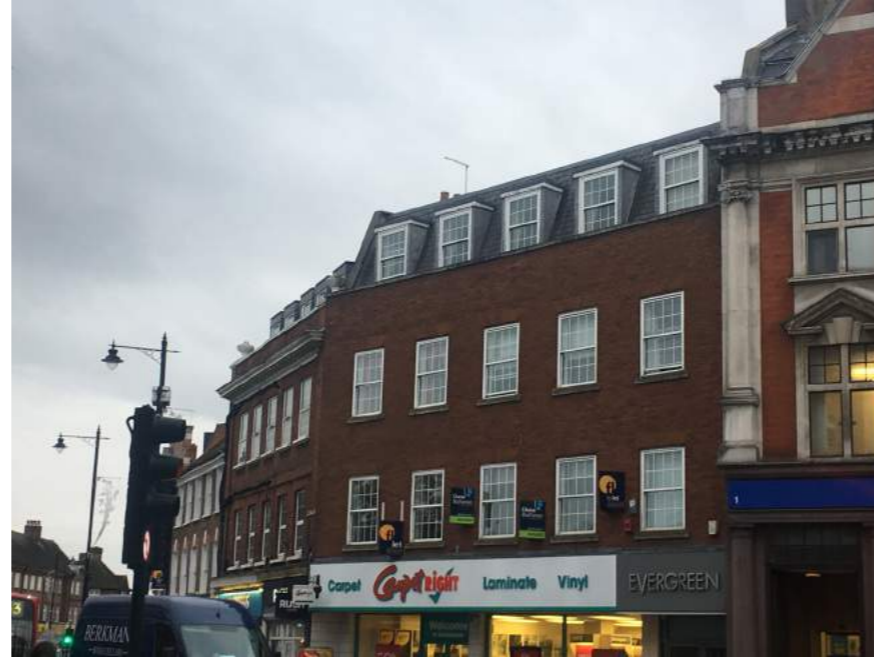
2. Mansard Roof and dormer windows - King Street
