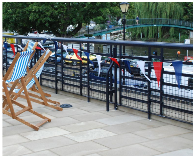
W2, Precedent - existing railing to DJG
