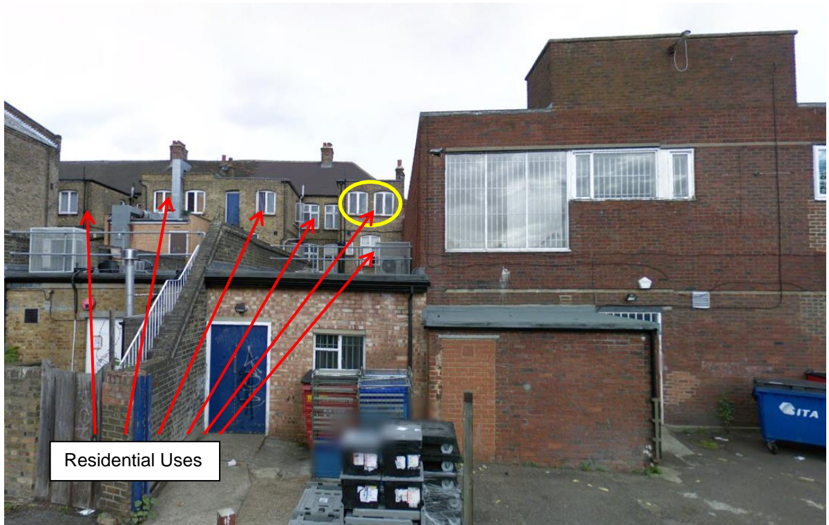
Figure 31: Service Road - Residential Uses
