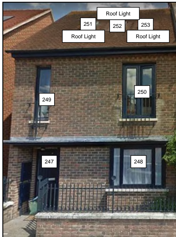
7 to 9 Water Lane
