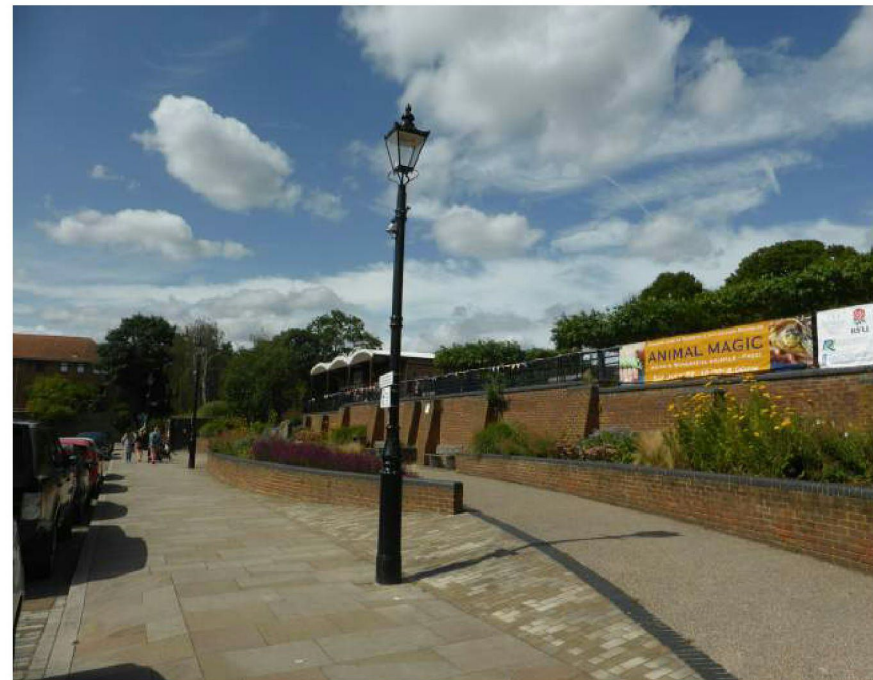
The front of the site connecting through steps to Diamond Jubilee Gardens
