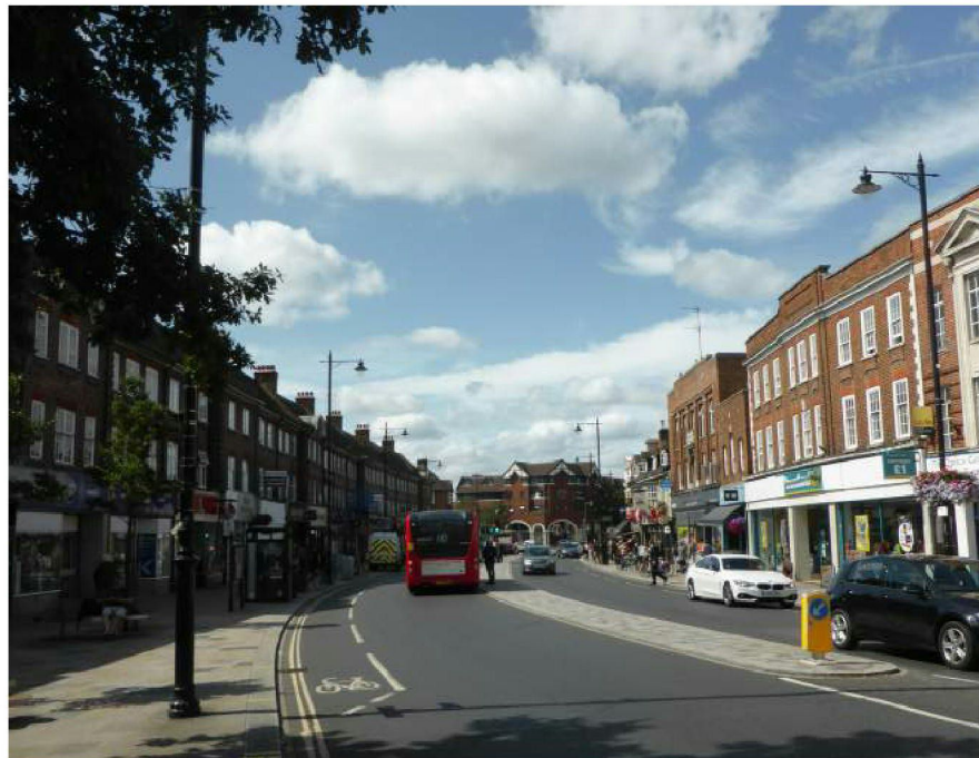
1. View looking west along King Street
