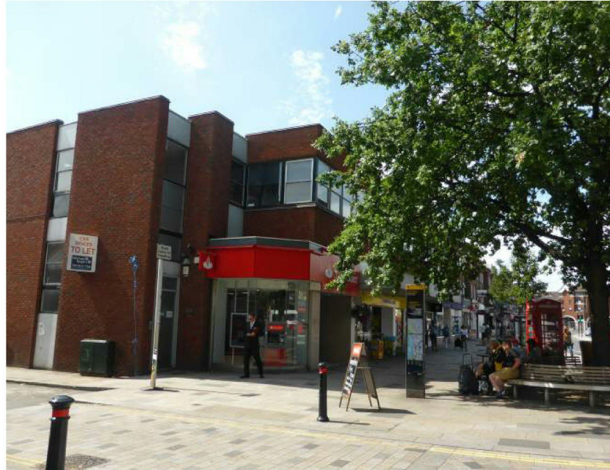
View looking south west towards the site (Santander & Superdrug)
