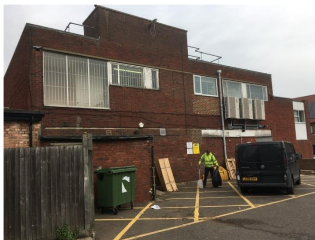
Rear elevation of the current holding fronting King Street
