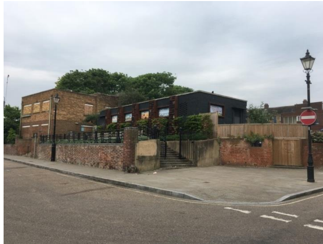
Looking north-west from the river at the disused buildings on site
