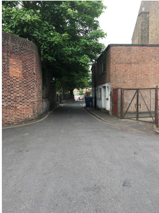
Looking west along current service road
