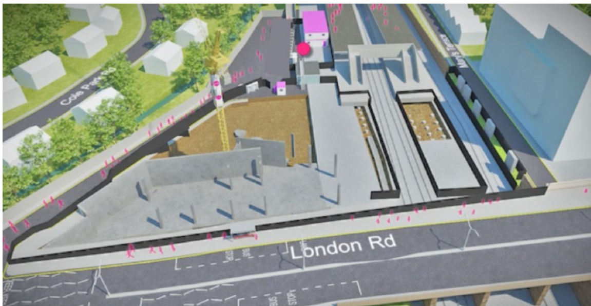
Figure 21: Block A Frame and Island Pile Caps
