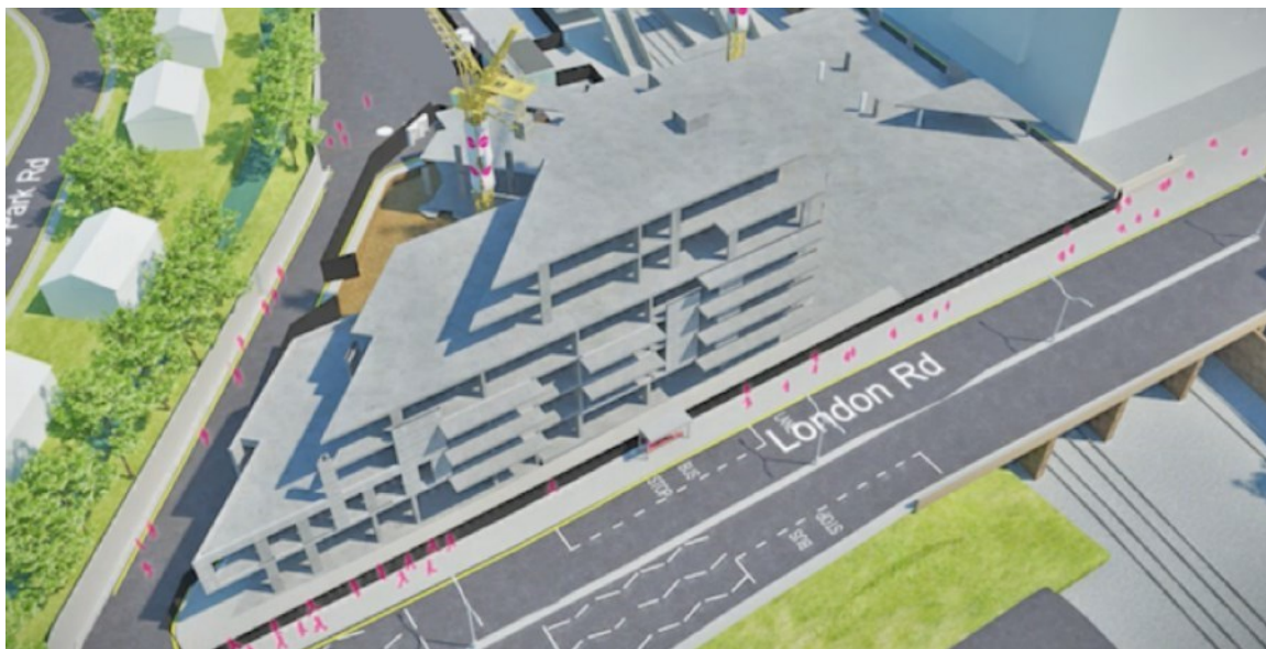
Figure 26: Deck Slab in Position
