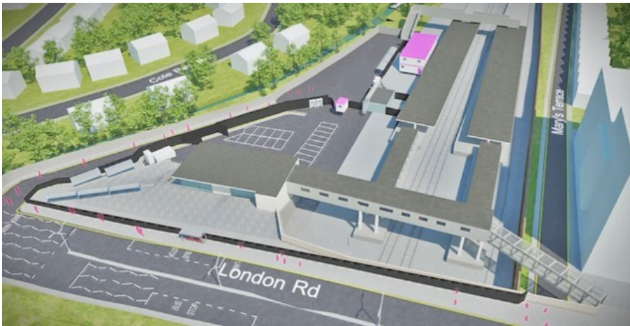
Figure 10: Site Establishment with new Temporary Ticket Office
