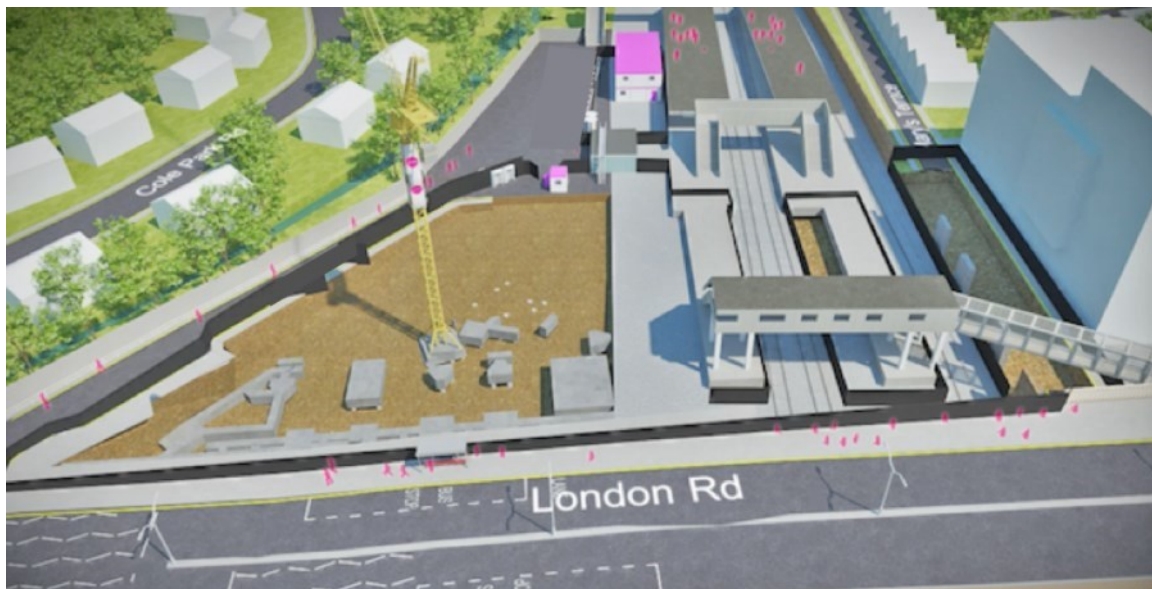
Figure 20: Block A pile caps piling – Tower crane and Mary's Terrace pile caps
