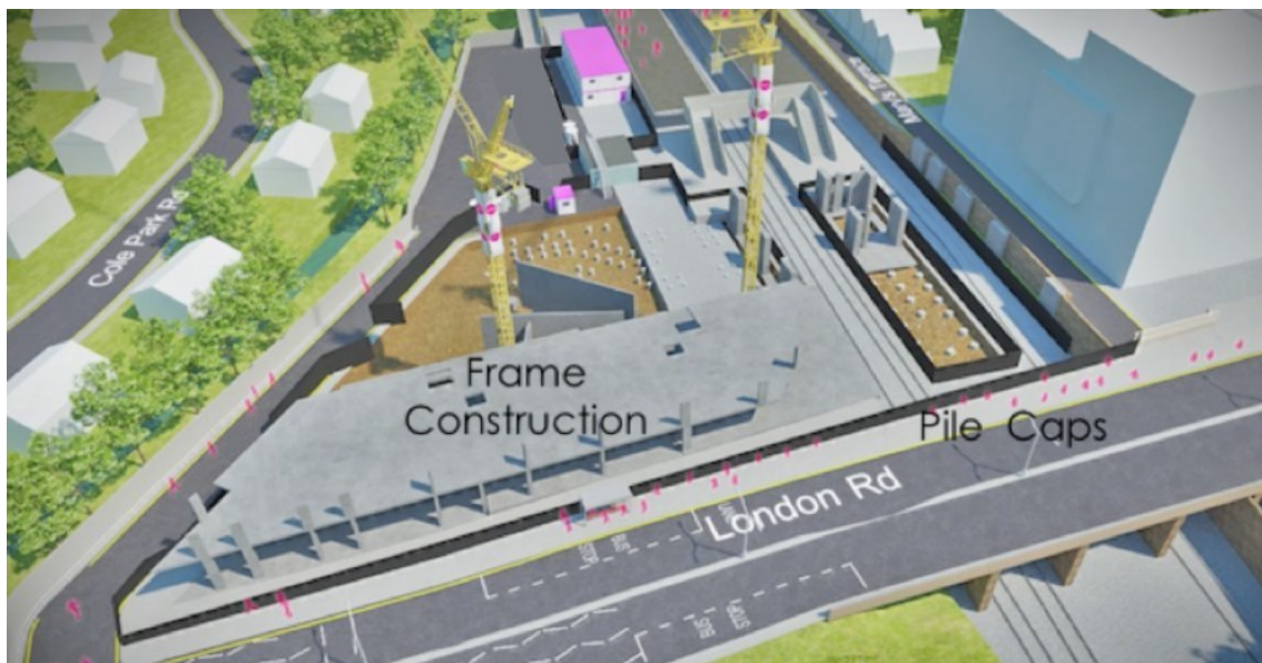
Figure 24: The First level of Post Tensioned Concrete Frame
