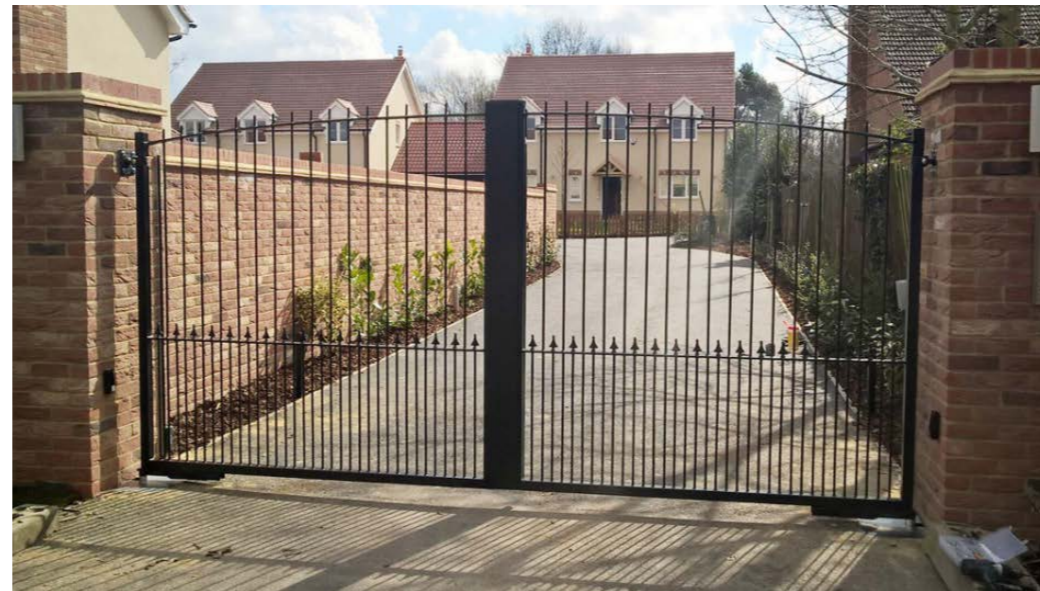
Steel double gate 1.8m
