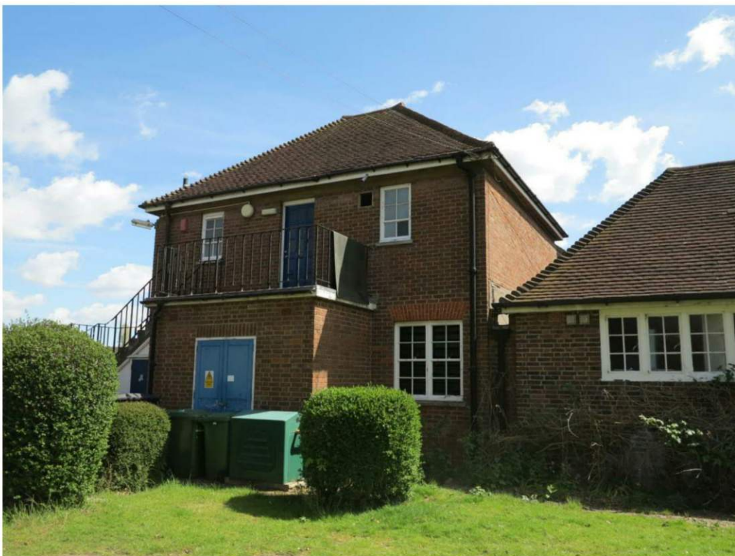
Plate 12. The eastern elevation of the 1960s' extension
