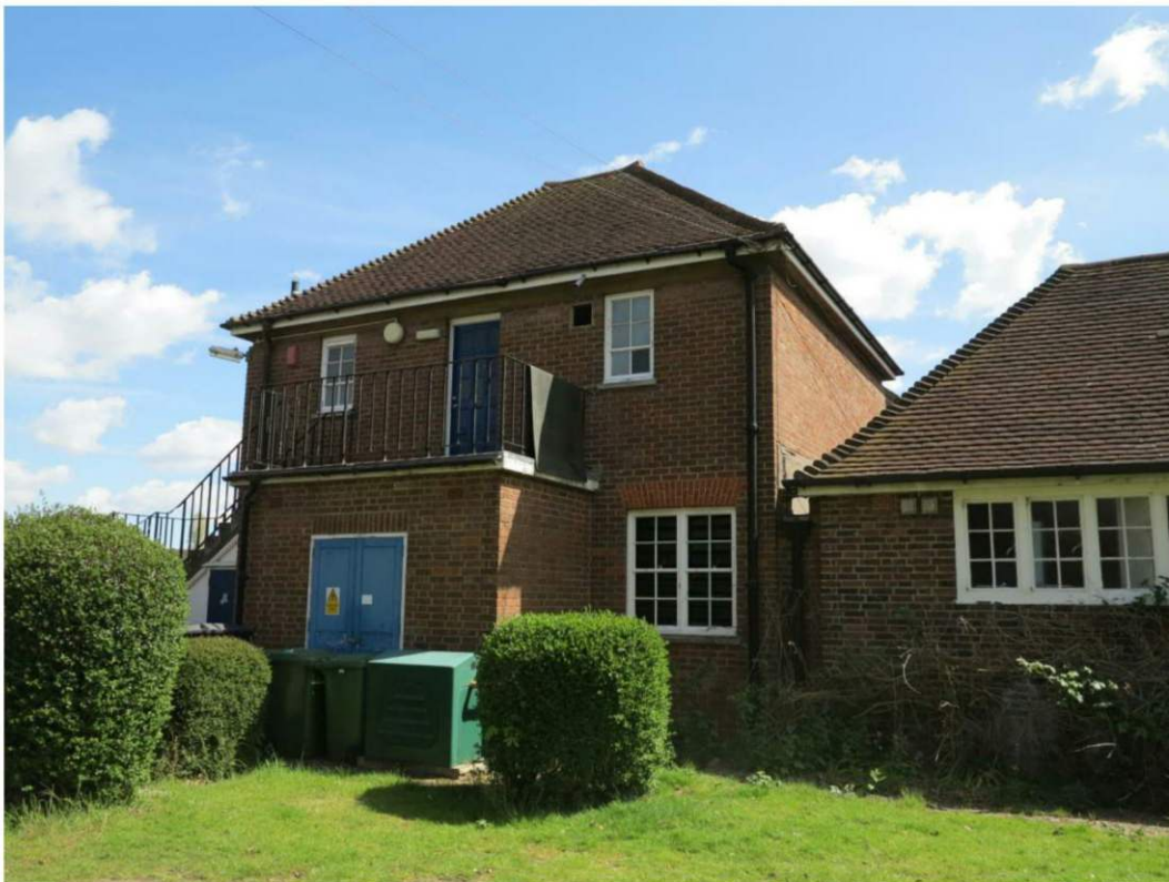
Plate 12. The eastern elevation of the 1960s' extension
