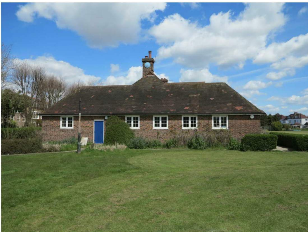
Plate 4. The southern elevation of the pavilion
