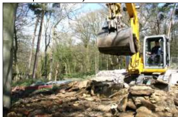
Hard surfacing/structure removal image 2: Machines with a long reach can be used to lift out heavy surfacing and structures as long as the machine sits outside the RPA and the exposed surface is protected before there is any further access.
