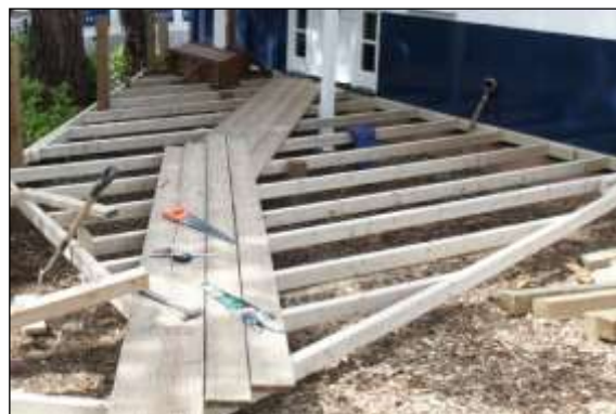
New structure image 2: This deck supported above the ground on small posts provides a low-impact alternative to conventional stone patio surfacing in RPAs.
