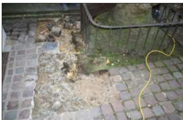
Hard surfacing/structure removal image 3: Careful lifting of cemented-in sets round this tree allowed them to be re-laid on a permeable sand base, improving the water input into the soil around the trunk.
