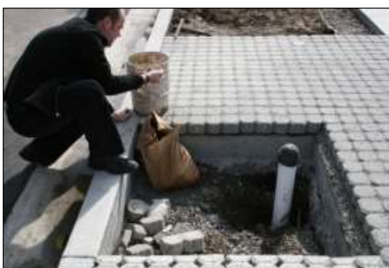
Soil cell image 3: The finished surfacing is profiled to leave the tree pit open, ready to be filled with good quality topsoil and the new tree.
