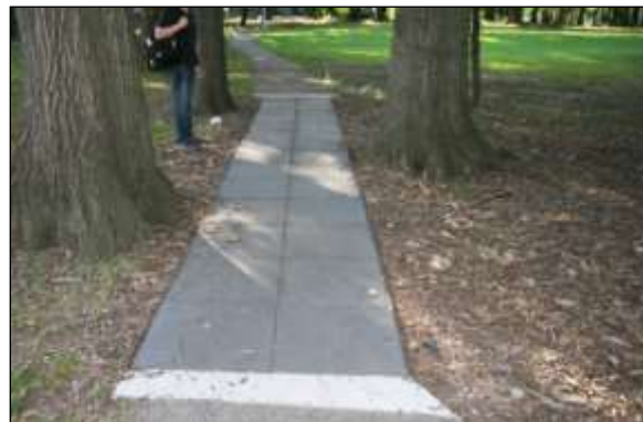
New surfacing image 11: Where surfacing is needed close to rapidly growing buttress roots, a light metal frame with rubberised surfacing will allow the path to distort without cracking as the roots grow.
