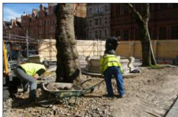
Hard surfacing/structure removal image 4: These trees had impermeable surfacing right up to their trunks, which had to be removed by hand before installing new structures.
