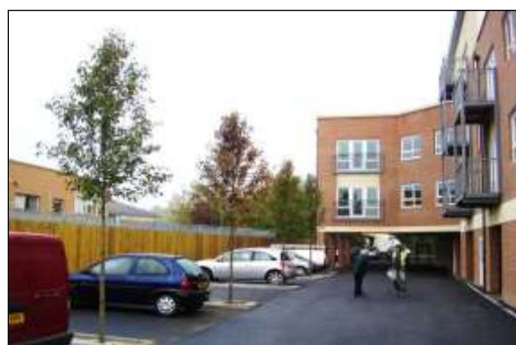
Structural soil image 2: It allows trees to be successfully established in areas of extensive hard surfacing, with very little, if any, loss of parking space.
