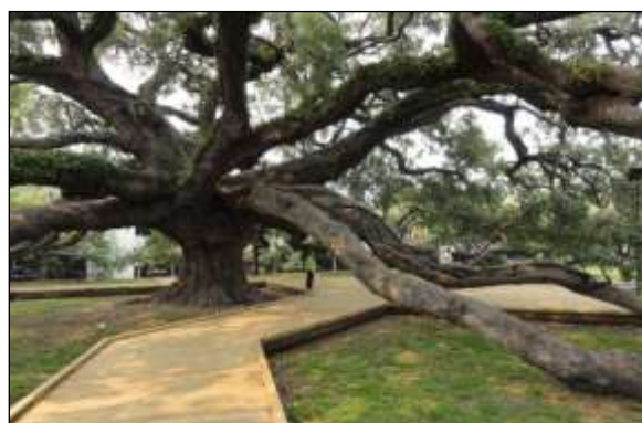
New surfacing image 9: Board walks supported on posts or a light frame are another way of providing pedestrian access across sensitive RPAs (photo courtesy of Philip van Wassenaer).
