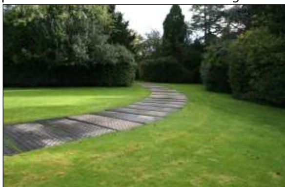
Hard surfacing/structure removal image 1: Ground protection must be used where repeated foot or vehicle traffic could cause compaction in sensitive RPAs. It can be as simple as plywood for pedestrians, but must be more robust for vehicles.
