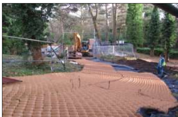
New surfacing image 2: The three-dimensional cells are opened up, spread across the area to be surfaced and pinned in place ready for the stone filling.
