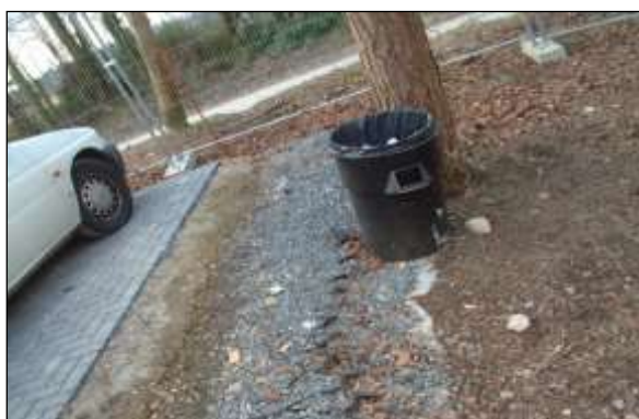
New surfacing image 4: A conventional concrete haunching can be used to retain new surfacing as long as it is not dug into a trench - here it is placed on top of the CellWeb layer.
