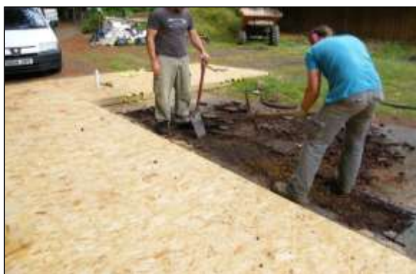
Excavation image 1: Careful hand-digging using conventional tools is acceptable for exposing roots in RPAs.
