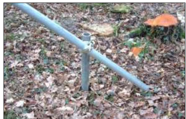
Fencing image 3: Close up of bracing detail, essential for increasing the stability of the vertical framework.
