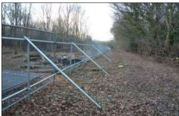
Fencing image 2: Heras fencing wired to scaffold braced posts is a robust and effective interpretation of the BS specification.
