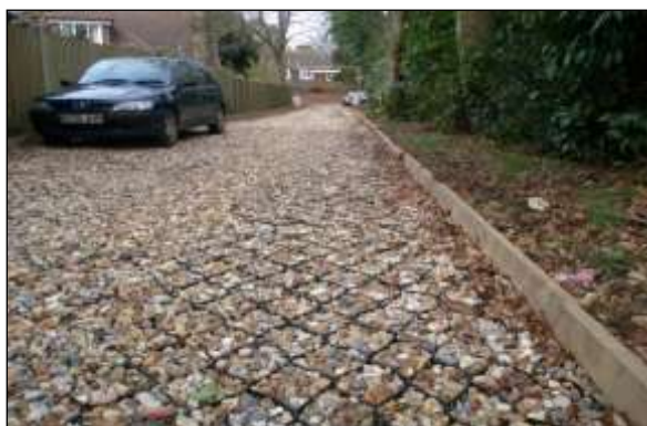
New surfacing image 6: Wooden board pinned in place or held in position with backfilled topsoil can provide more informal and rustic surface edging.
