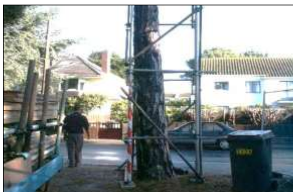
Fencing image 5: A scaffold-braced framework surrounding the trunk reduces the risk of accidental impact.
