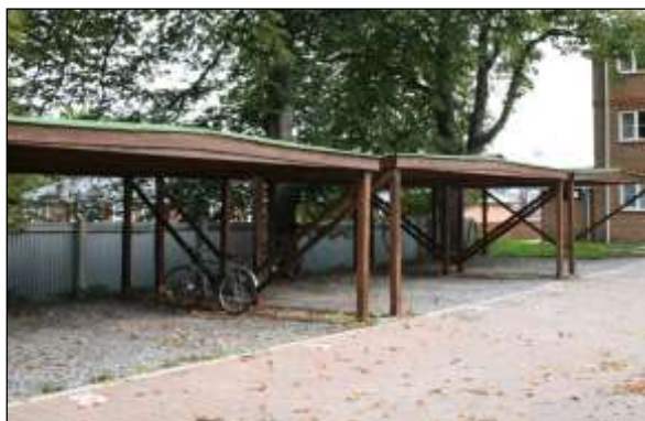
New structure image 1: These carports are formed by wooden posts above a three dimensional cellular no-dig and load-spreading surface of permeable crushed stone.
