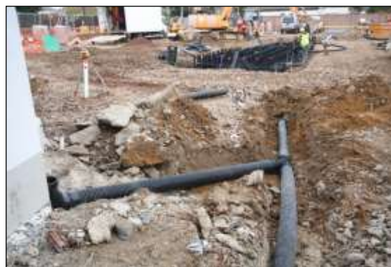
Soil cell image 2: Drainage from adjacent buildings can be directed into Silva Cells, significantly buffering rainwater runoff from urbanised areas.
