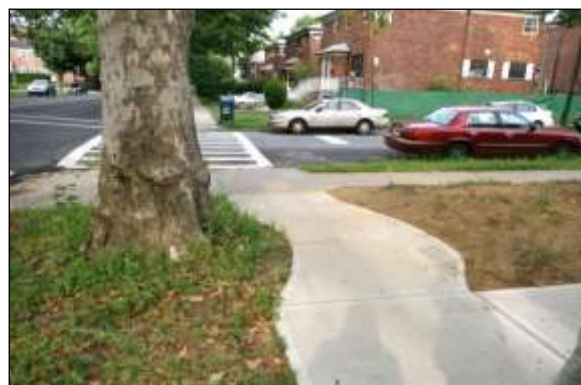
New surfacing image 7: In some situations, it may be appropriate to cast a free floating concrete surface directly onto the soil surface provided provision is made to prevent soil contamination while the concrete is being poured, i.e. an impermeable membrane separating the concrete from the soil.
