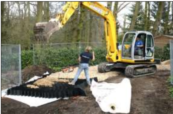
Ground protection image 5: Cellular products are a very effective means of providing ground protection where heavy vehicle use is expected. Here, it is being used to temporarily widen an existing road, to be removed once the construction is finished.
