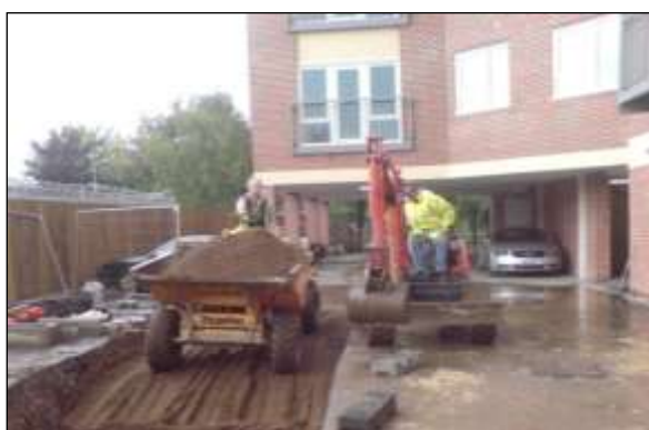
Structural soil image 1: Structural tree soil retains sufficient structure for tree roots to grow, even when compacted.
