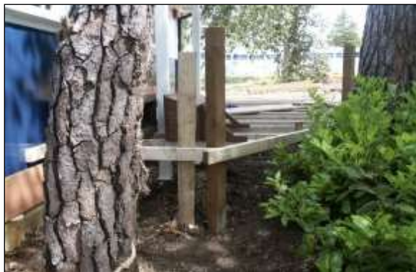
New surfacing image 10: New surfacing can be supported above the ground on posts leaving the soil surface beneath undisturbed.
