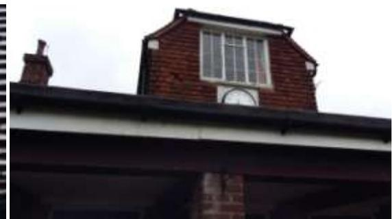
Missing hanging tiles providing bat access
