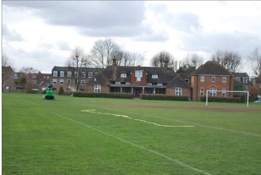
Plate 2: General view of pavilion building at west of site, looking west
