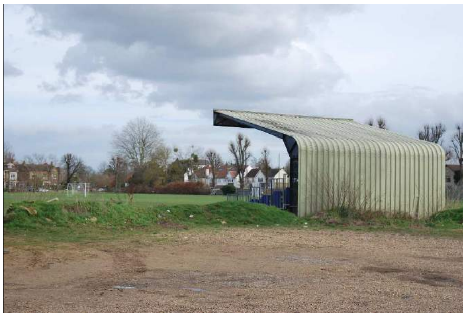
Plate 3: Metal spectator stand at west of site, looking southeast
