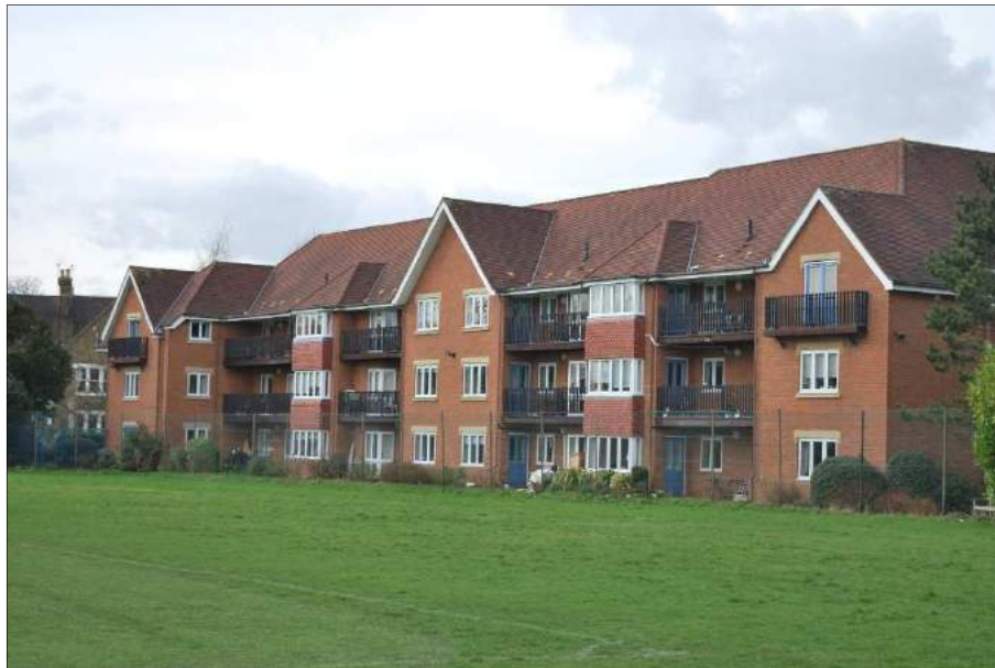
Plate 5: Residential flats bordering the north of site, looking northwest
