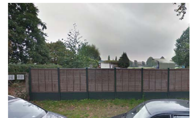
6 - Udney Park Road - Timber panelled boundary wall & grass verge
