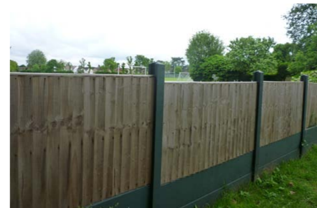
5 - Udney Park Road - Timber panelled boundary wall
