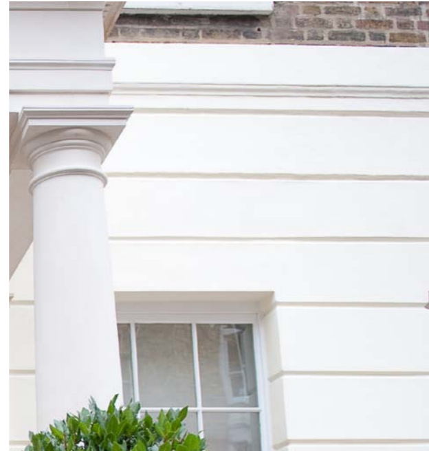
2. Smooth finished render with horizontal grooves
