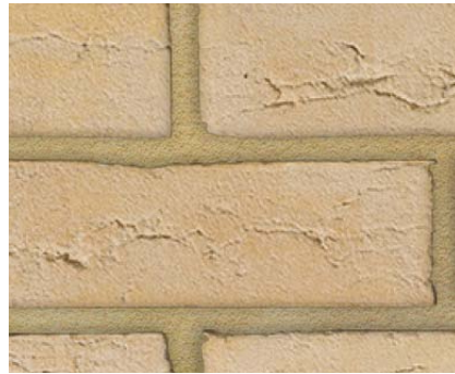
1. Face brickwork with sand colour mortar
