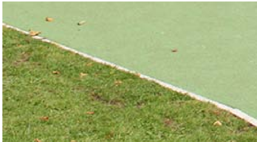
Outdoor Gym Rubber Safety Surfacing
