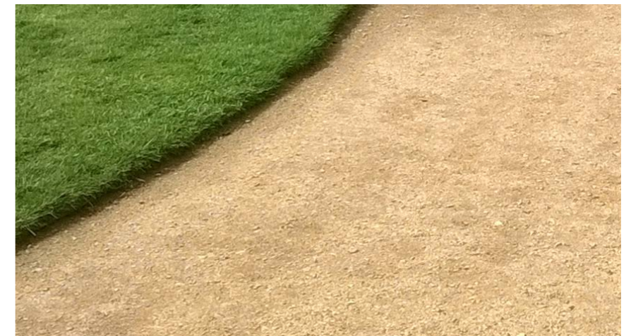
Self Binding Gravel Path
