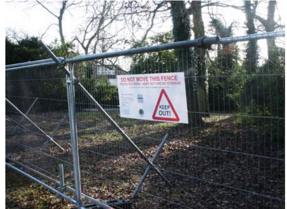
Effective fencing in position
