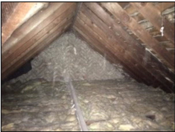
Image 14: Section of roof void over the gable addition to the house.
