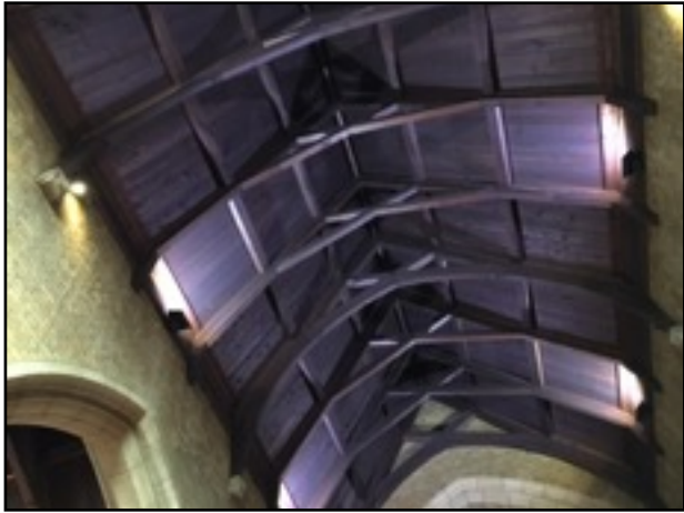
Image 10: Internal rafters of the church.
