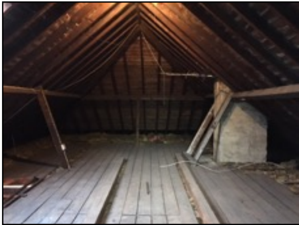
Image 12: Internal roof void of the bungalow.
