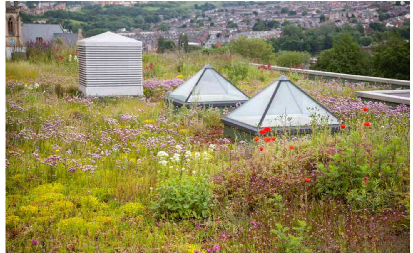
Non-intensive inaccessible green roof
