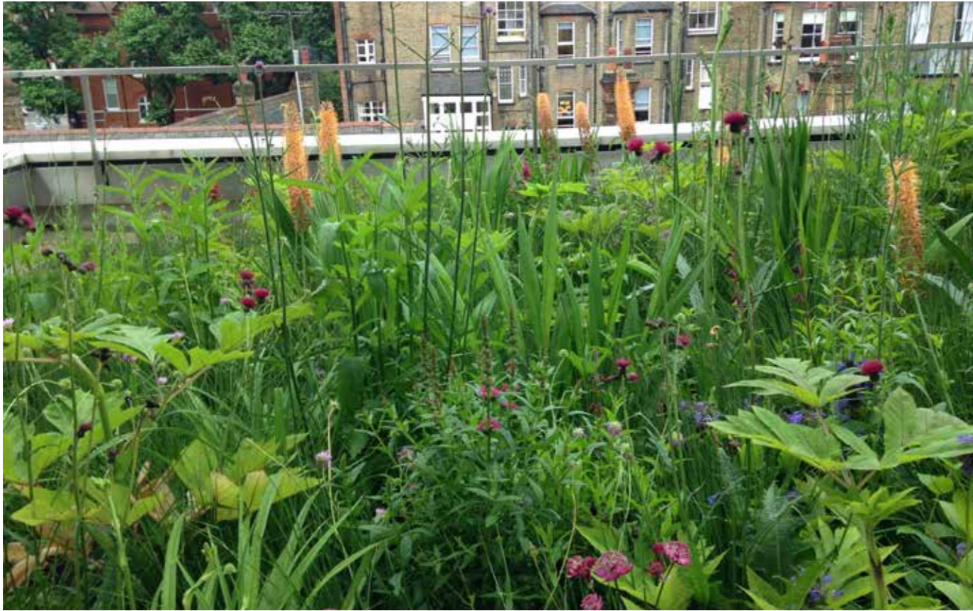
Intensive planting for accessible roof terraces
