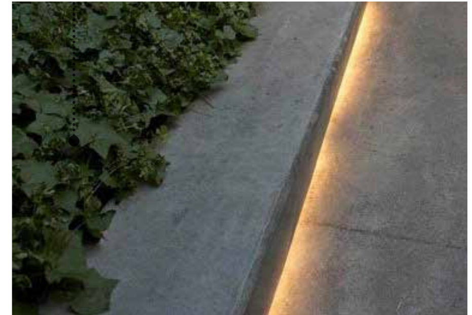
Light fittings integrated into a raised planter edge
