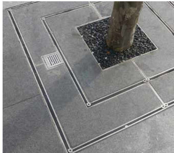
Granite slabs, tree pit detail
