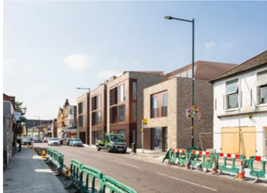
2. High Street Looking South
