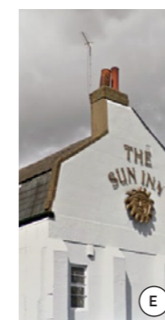
Irregular roof profile to neighbouring listed building
