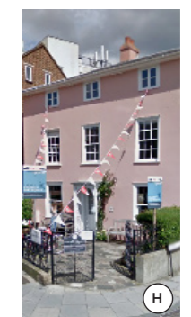
Grade II listed three storey building featuring hipped slate roof and square headed sash windows.
