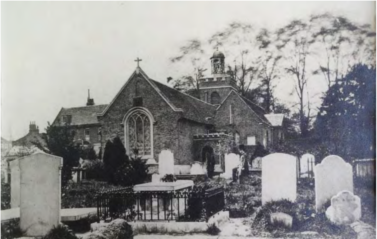
St Mary's seen from the east, probably in the 1860s/1870s: the chancel has been lengthened, but no tracery has yet been inserted in the windows of the 1753 north aisle. Church House is visible in the background. (London Borough of Richmond local studies library)
