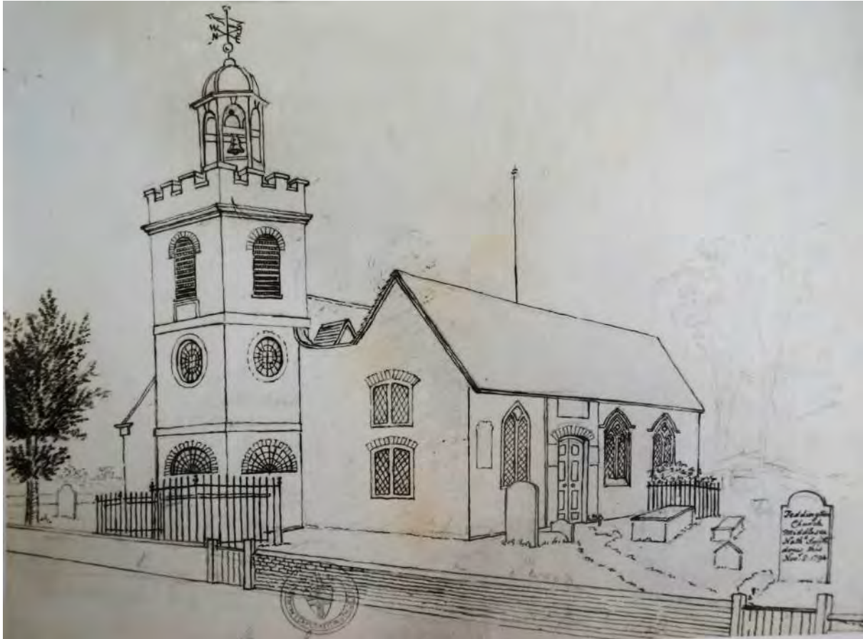
St Mary's from the southwest in 1794, pen drawing by Nathaniel Smith: the segmental-headed windows with a central mullion mark extension to the south aisle added by Hales; the upper one lit the gallery. (London Borough of Richmond local studies library)
