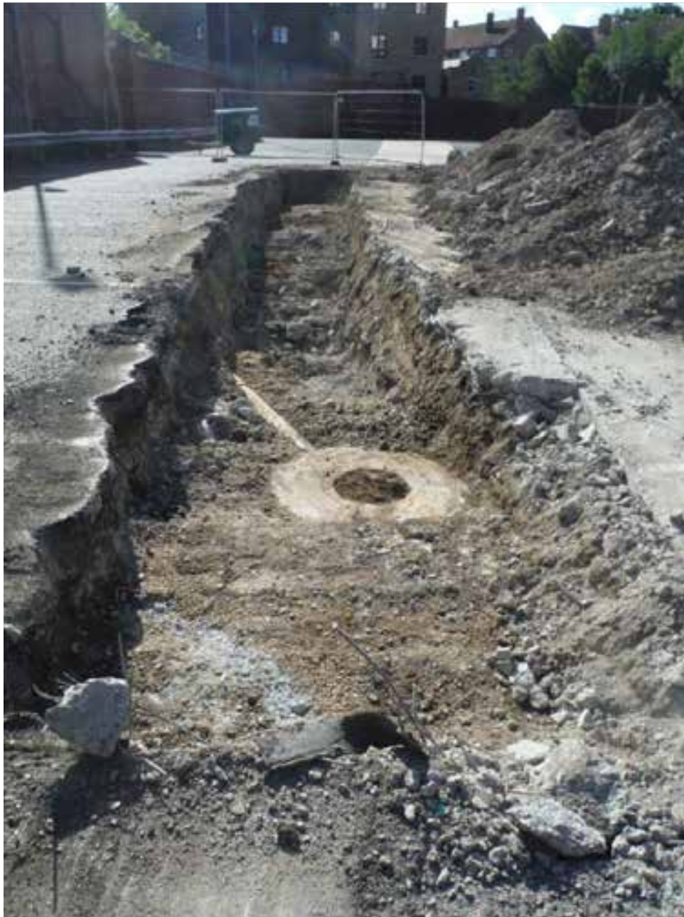
Image 8: East facing view of Trench 6
