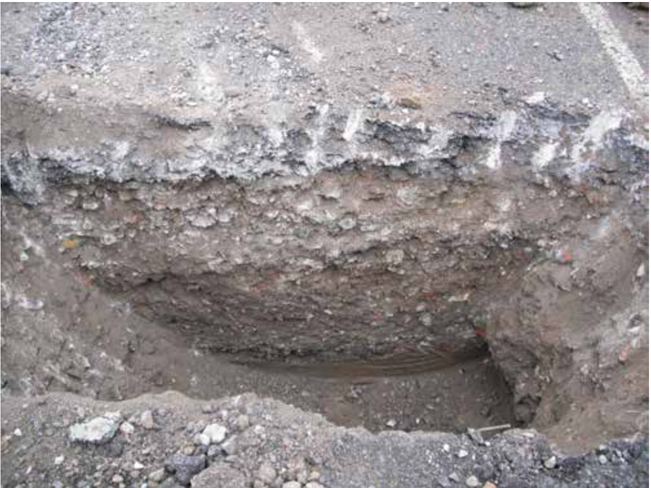
Image 13: North facing view of WS11 Sondage
