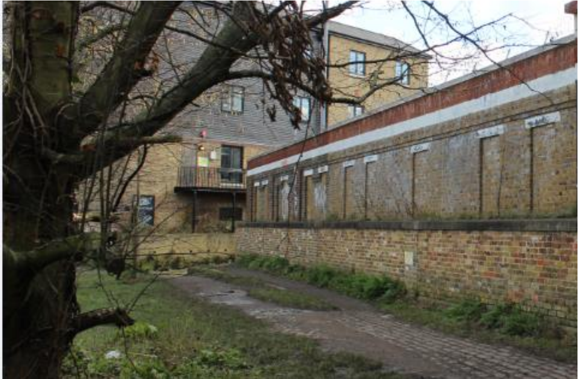
Figure 40: Sections 6 and 7 of the northern wall
