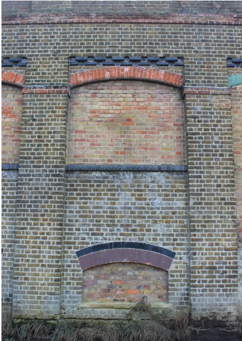
Figure 37: Part of the wall in Section 4.
