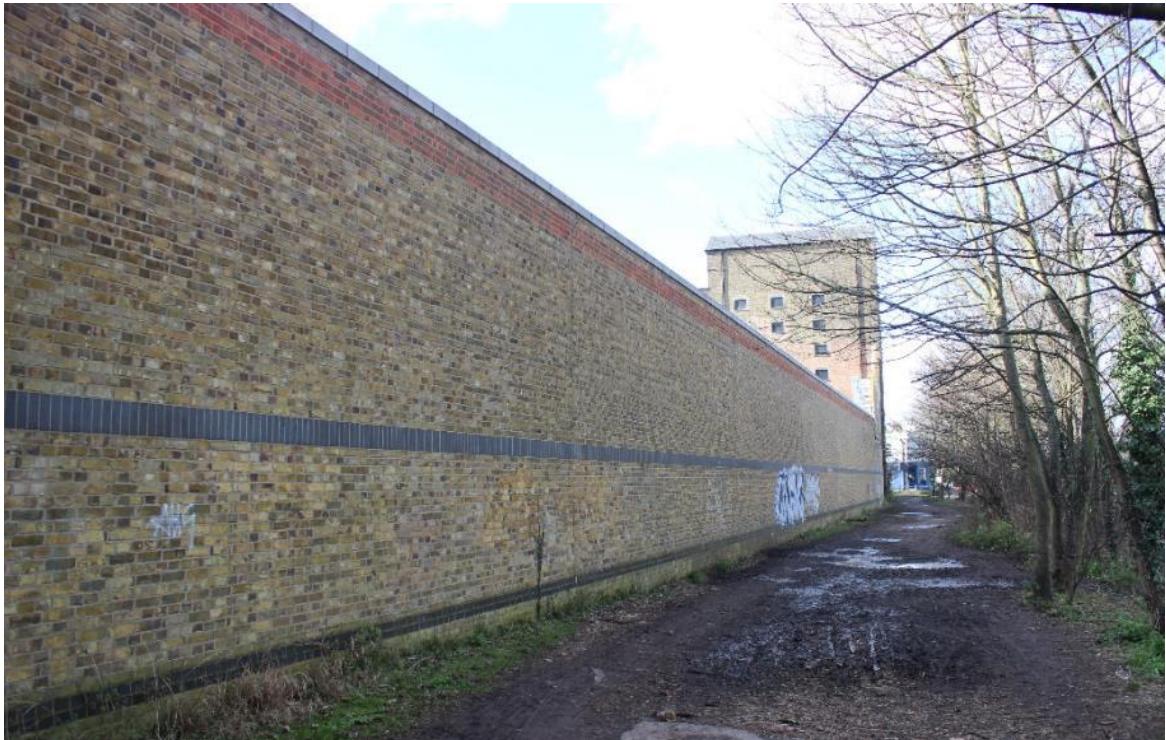
Figure 34: Section 1 - Late twentieth century wall.
