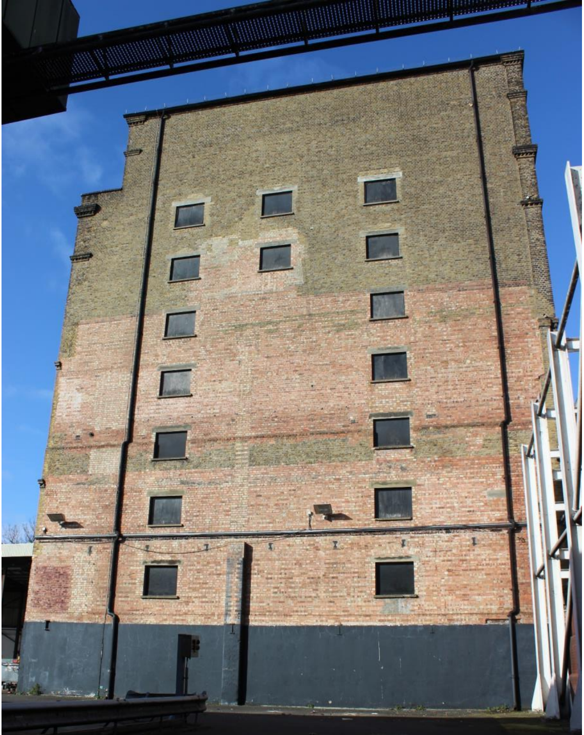
Figure 31: East facing elevation of Maltings
