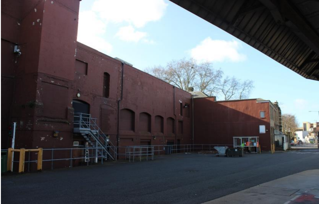
Figure 24: Northern, internal elevation of the former Bottling building
