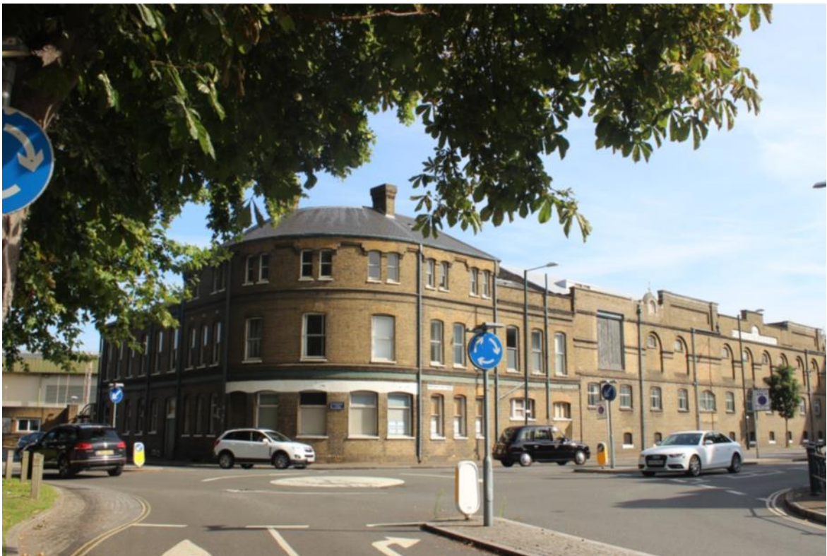
Figure 20: External, bowed, elevation of Former Hotel, facing onto the roundabout.
