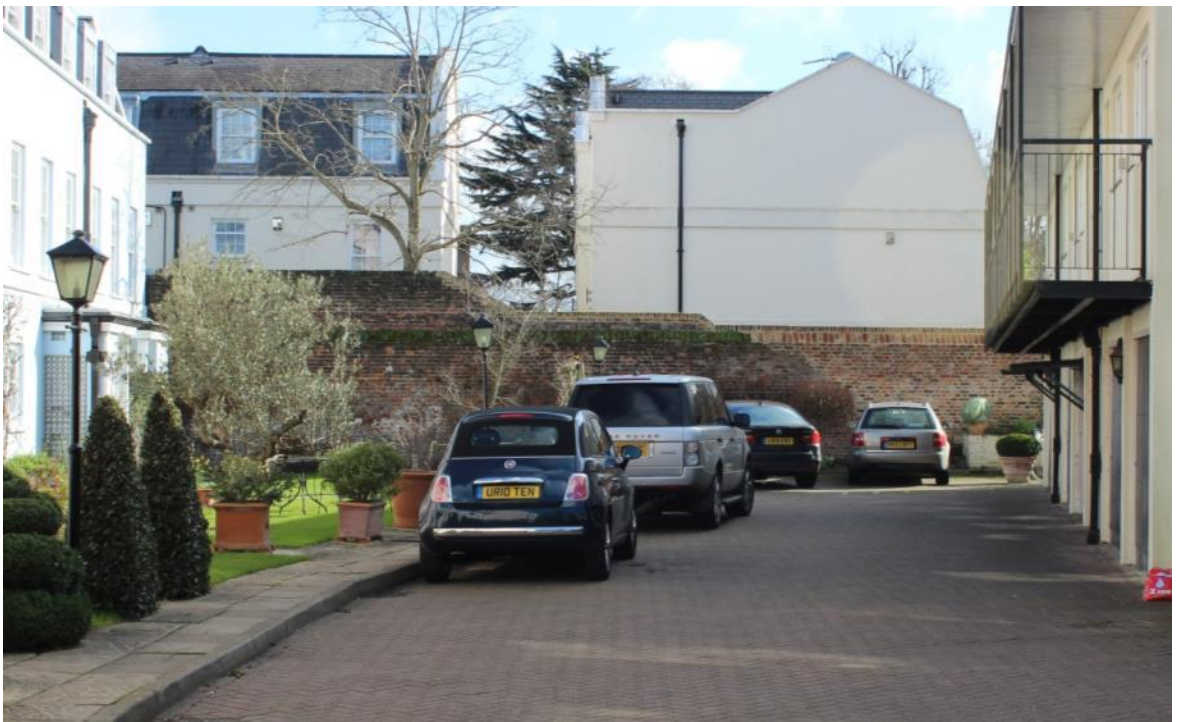
Figure 58: Garden Wall to east of Number 1-8 Riverside House
