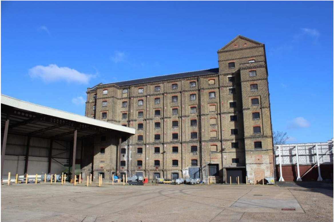
Figure 29: South facing elevation of Maltings.
