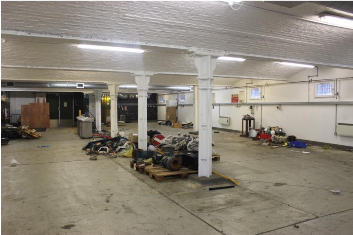
Figure 25: Interior of sub-ground floor of former Bottling building, illustrating brick arches and cast iron columns
