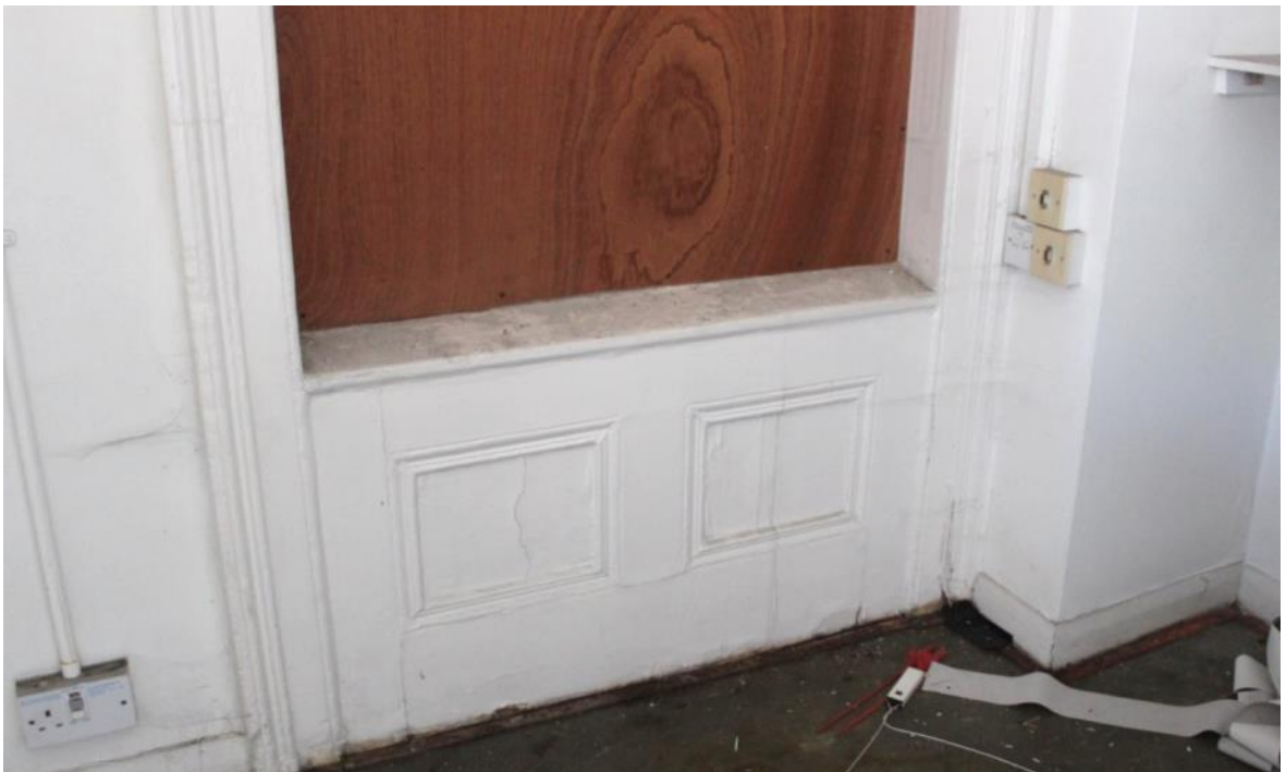
Figure 22: Surviving timber panelling to interior of Former Hotel
