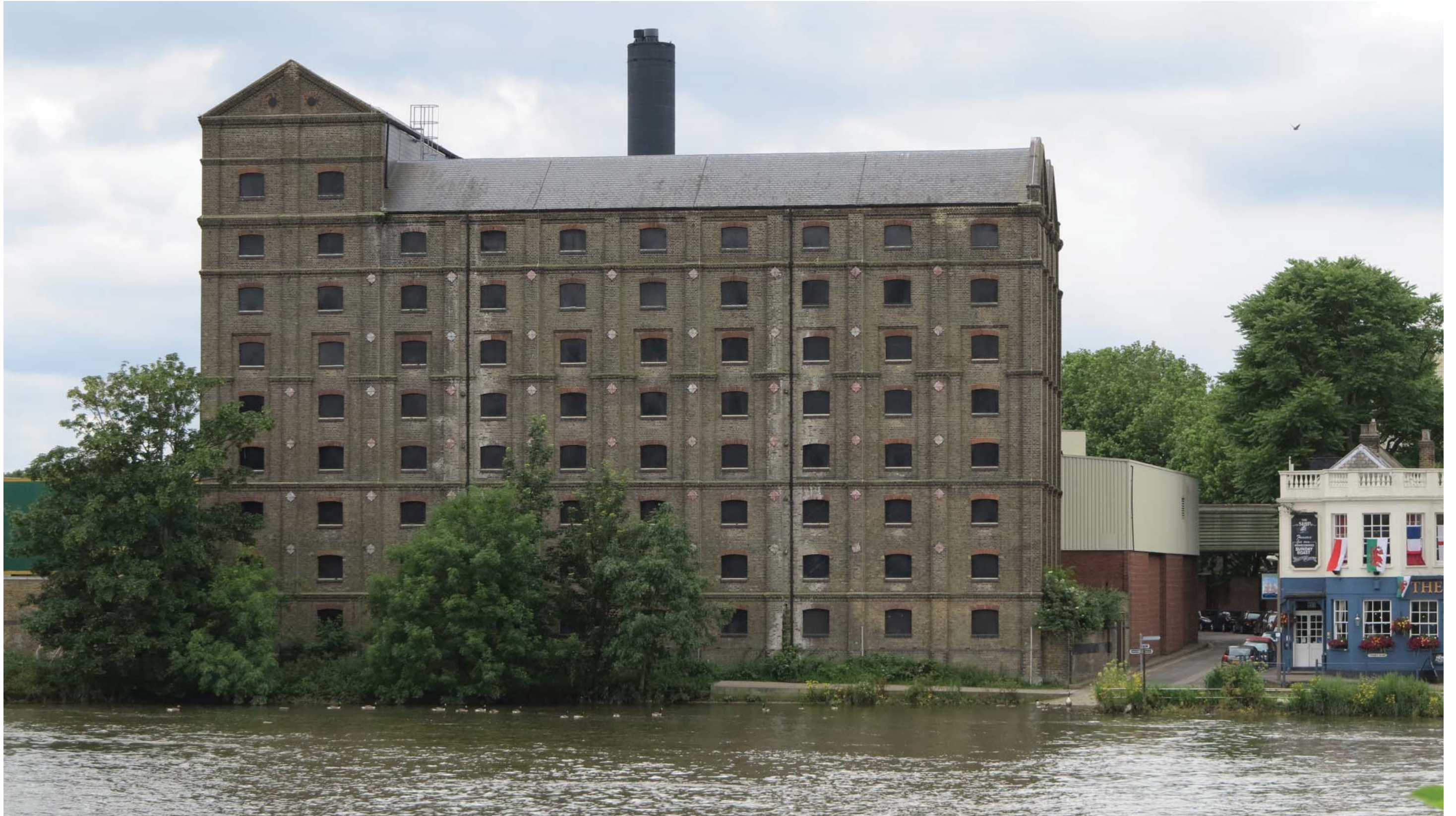
Photograph of existing Maltings building - North facade
