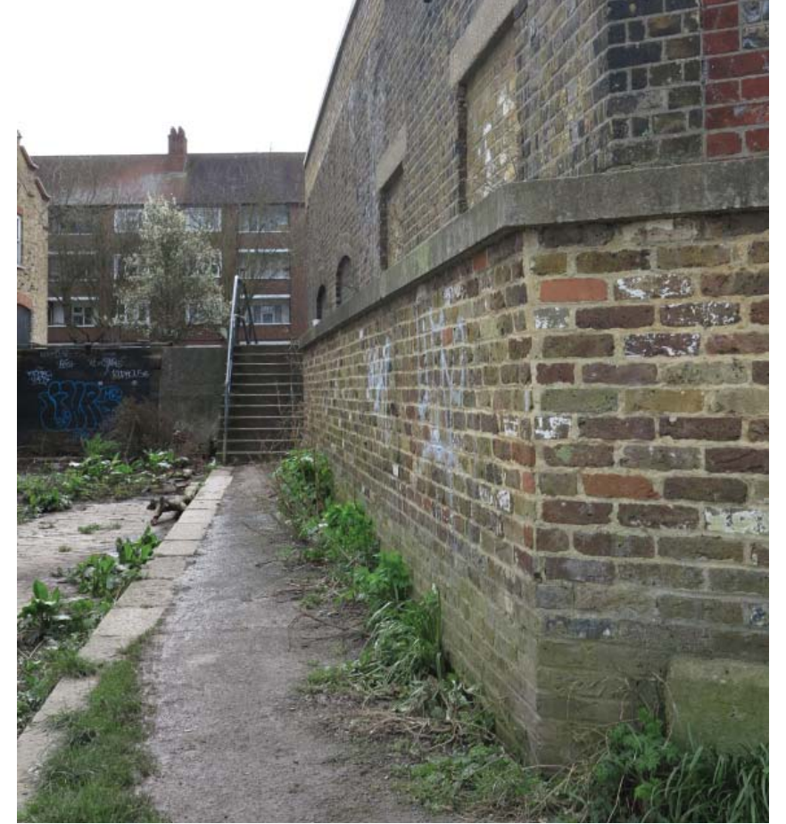
Photograph of existing Eastern boundary wall - towards Mortlake High Street
