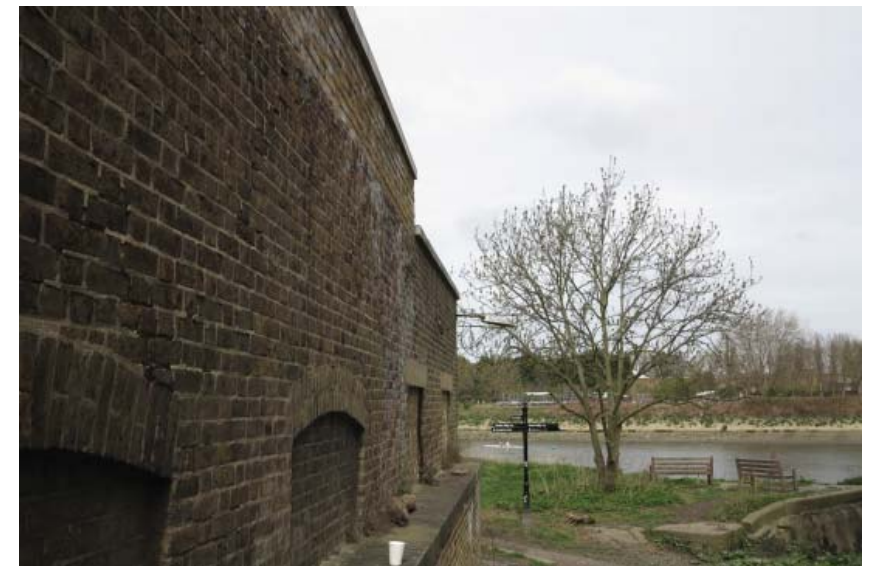
Photograph of existing Eastern boundary wall - adjacent to slipway
