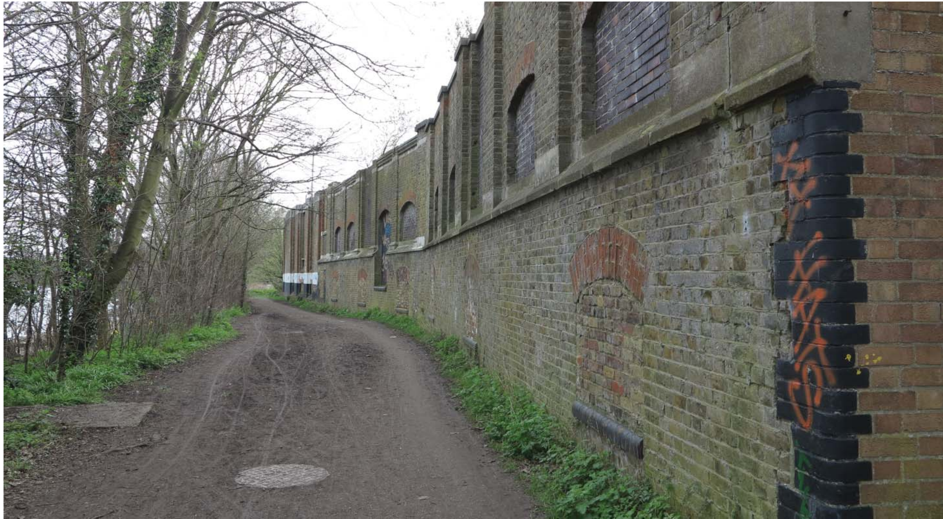
Photograph of existing Northern boundary wall
