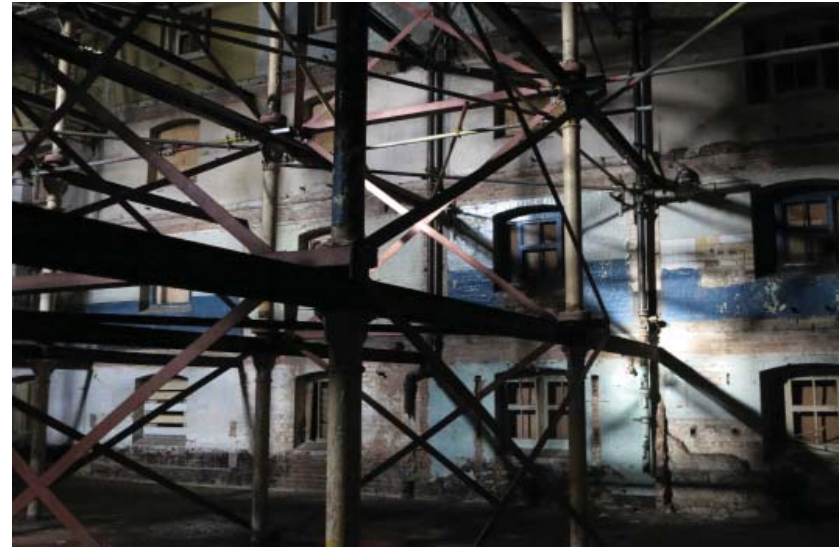
Photograph of existing Maltings building interior
