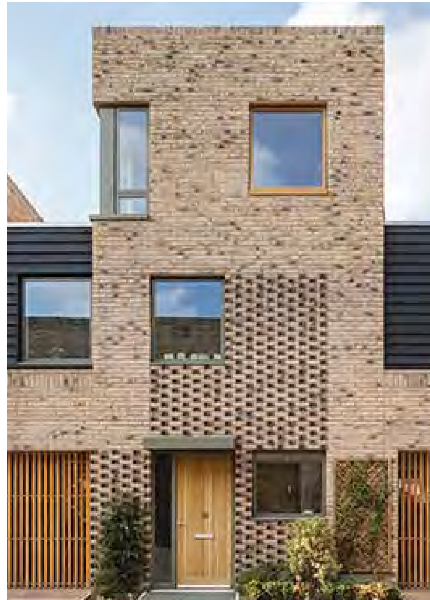
Example of timbers secondary elements only
