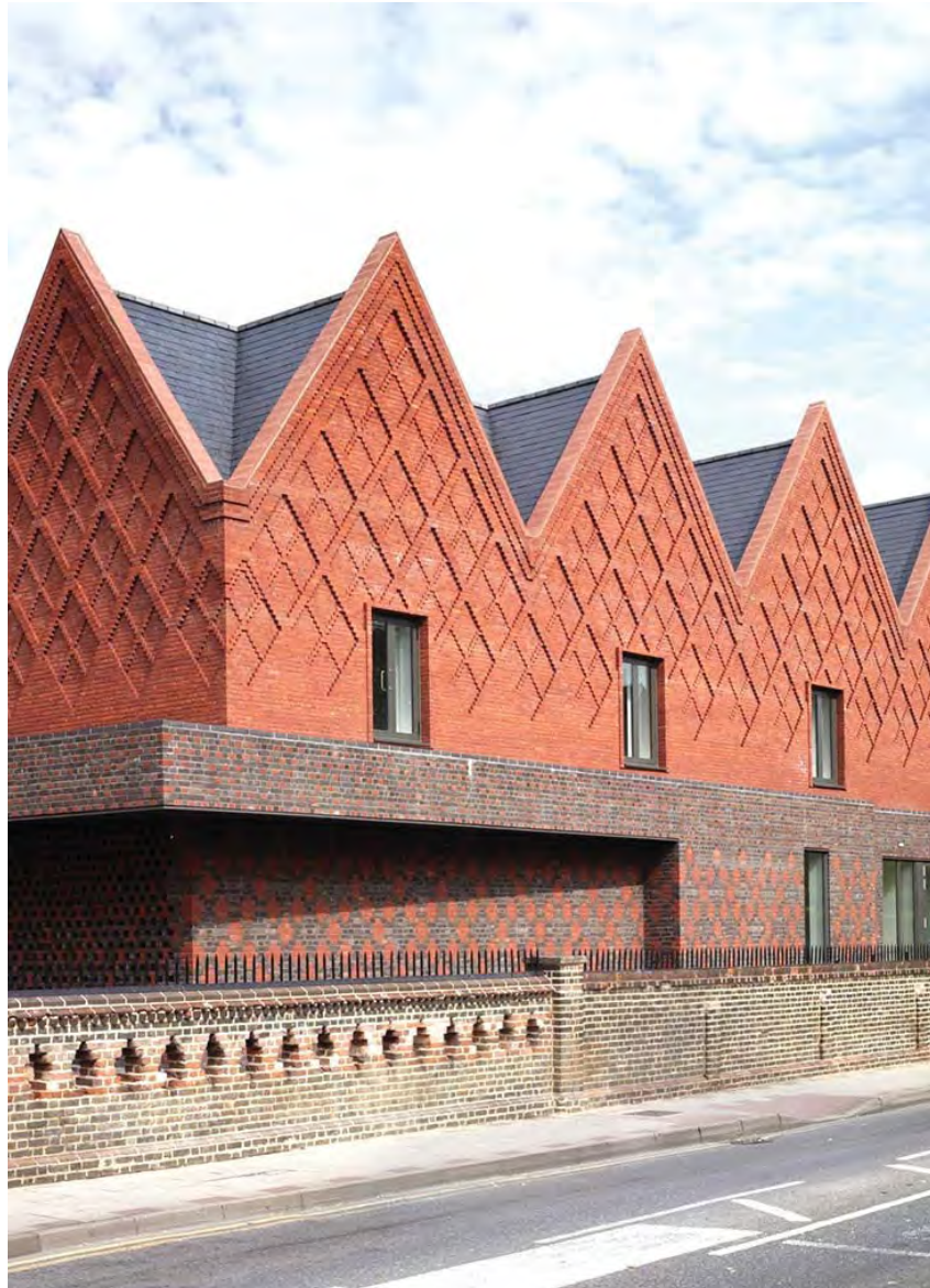
Example of contemporary detailing of vernacular form
