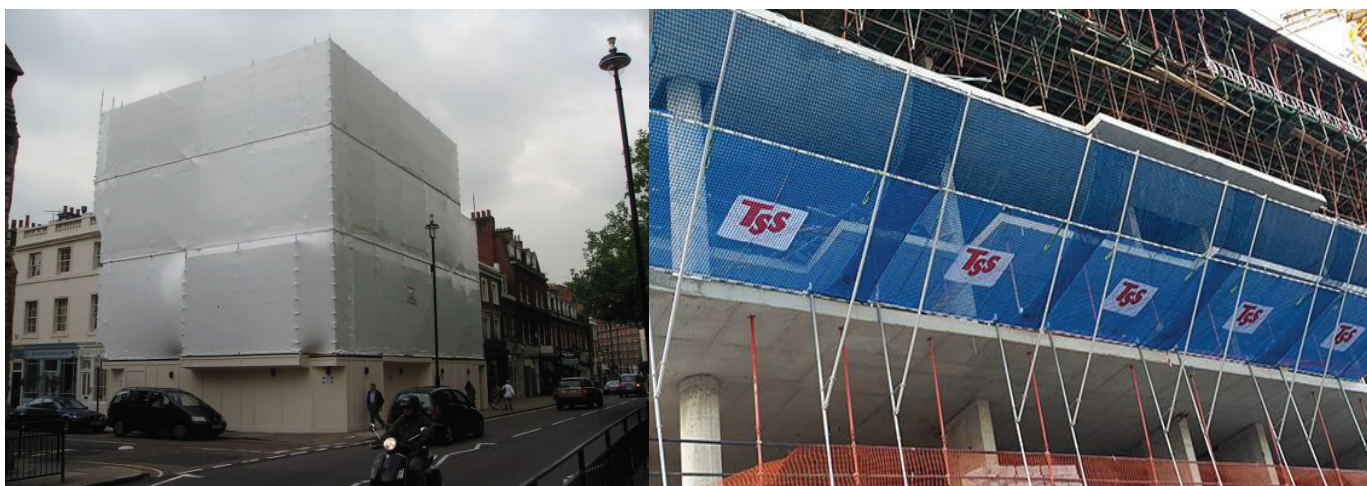
Figures 11 & 12: Full Building Scaffolding and Safety Fans
