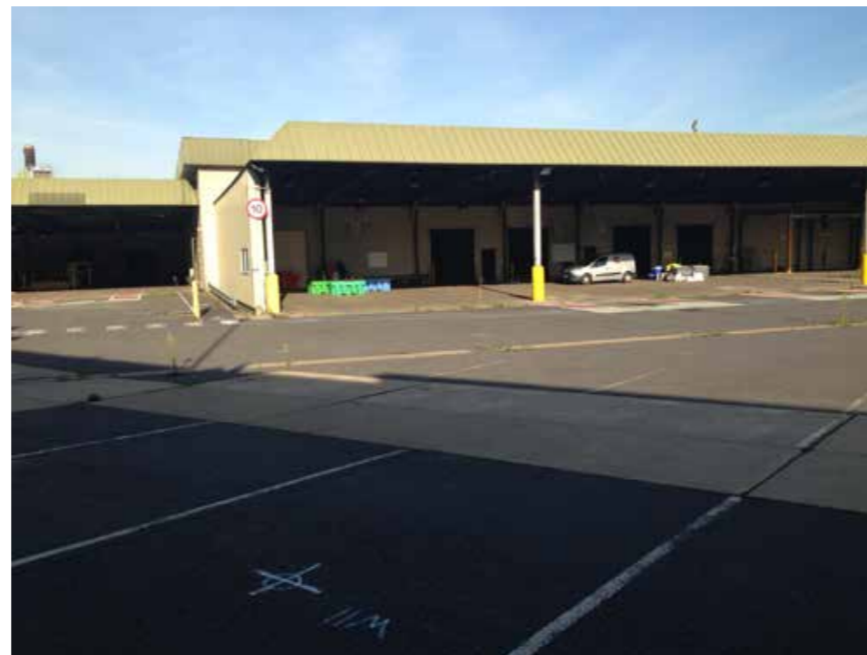
Photograph 5. General conditions at East Site
