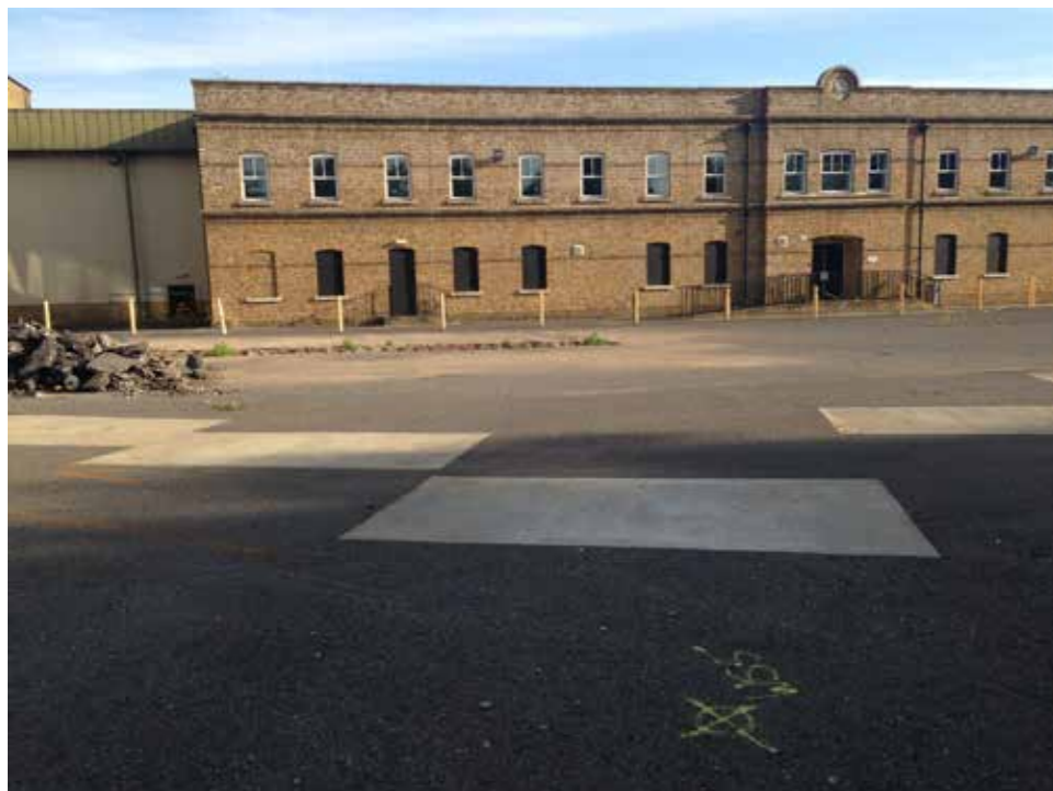
Photograph 4. General conditions at East Site
