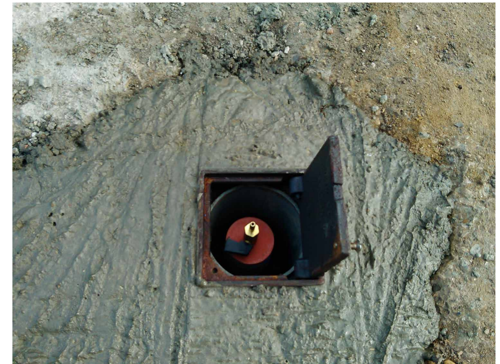
Photograph 8. Typical completed borehole
