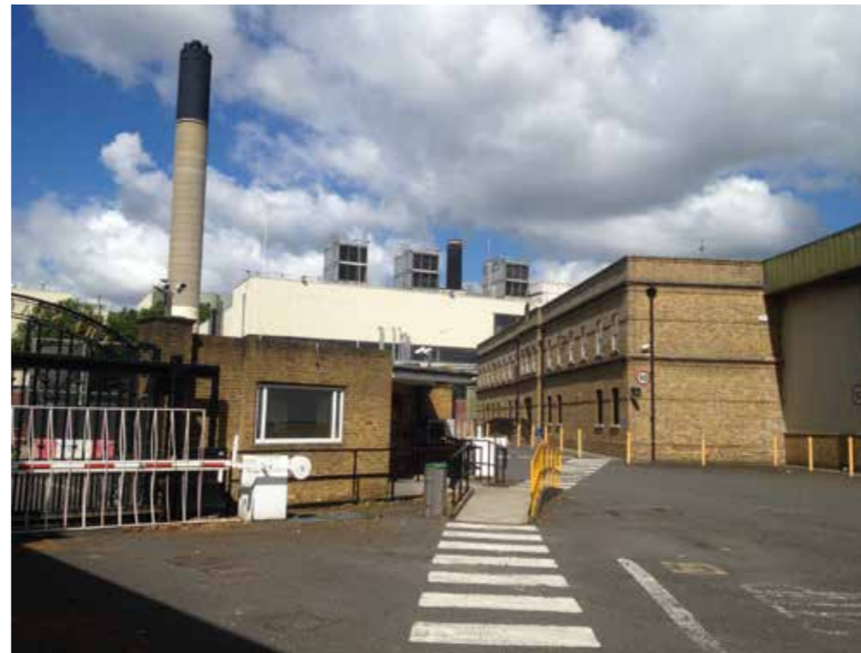
Photograph 2. General conditions at East Site
