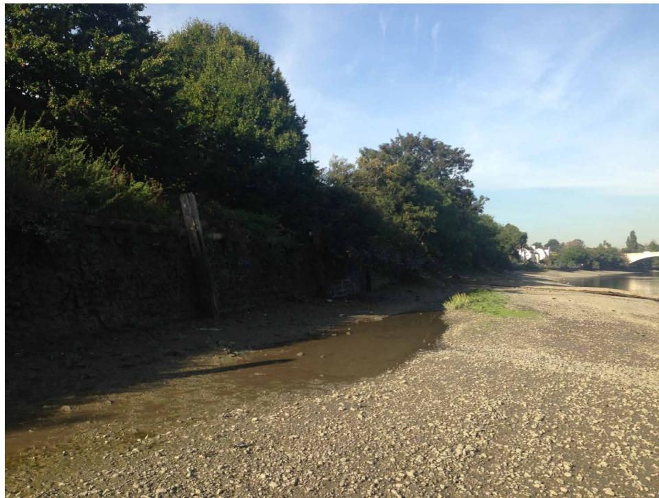
Photograph 6. General condition of River Wall adjacent to the Site
