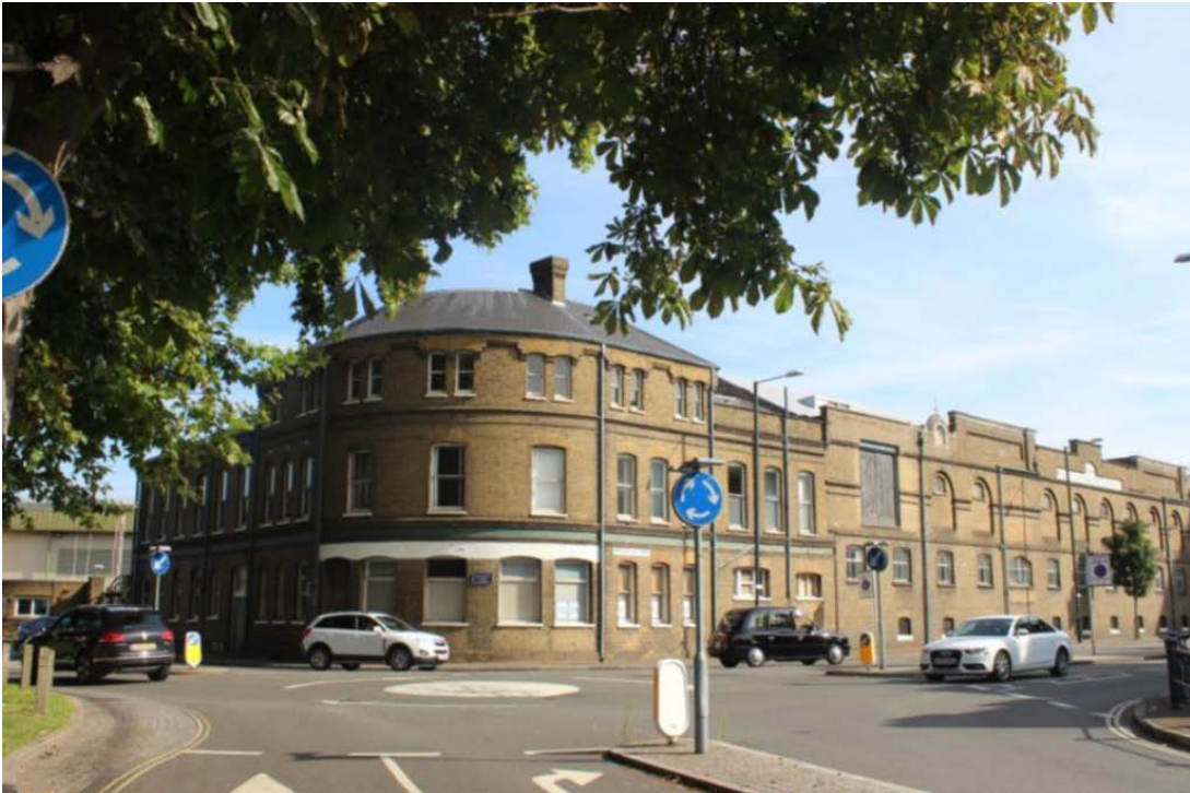
Former Hotel Building
