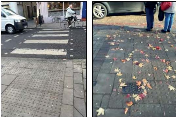
Figure 3.3: Crossings on Sheen Lane
