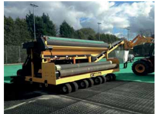
Automatic carpet lifting and rolling operation
