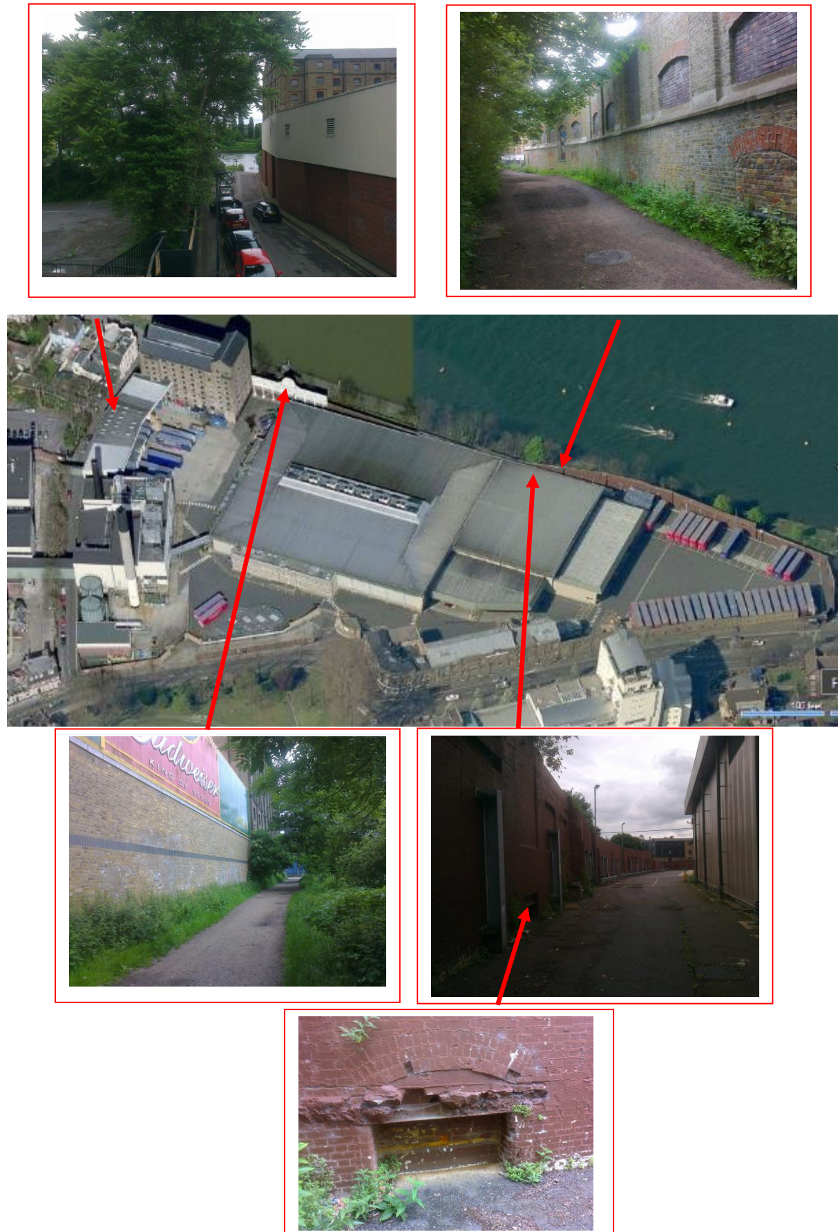
Figure 4-4 The extent of existing tidal defences
