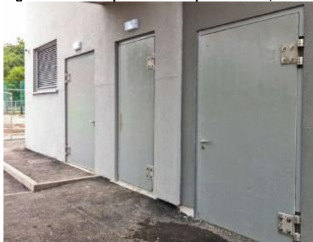
Figure 4-13 Examples of flood proof doors, suitable for sub-station facility
