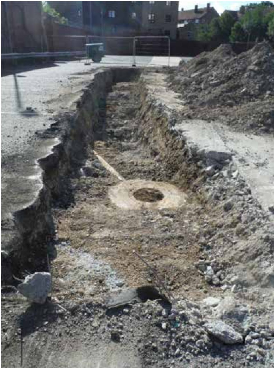
Image 8: East facing view of Trench 6
