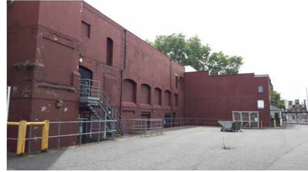
Photo 4 Former Hotel and Former Bottling Hall
