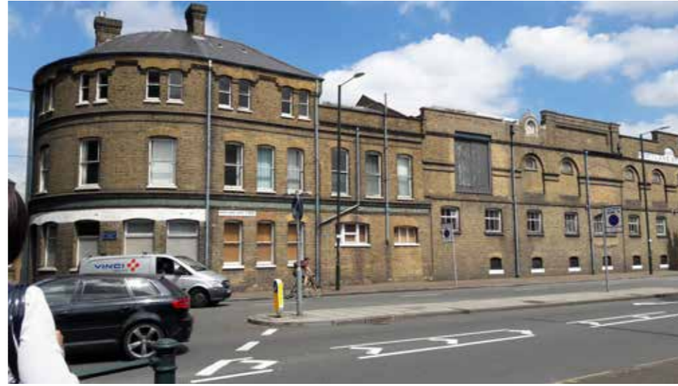
Photo 3 View of Former Hotel and Former Bottling Hall from Mortlake High Street
