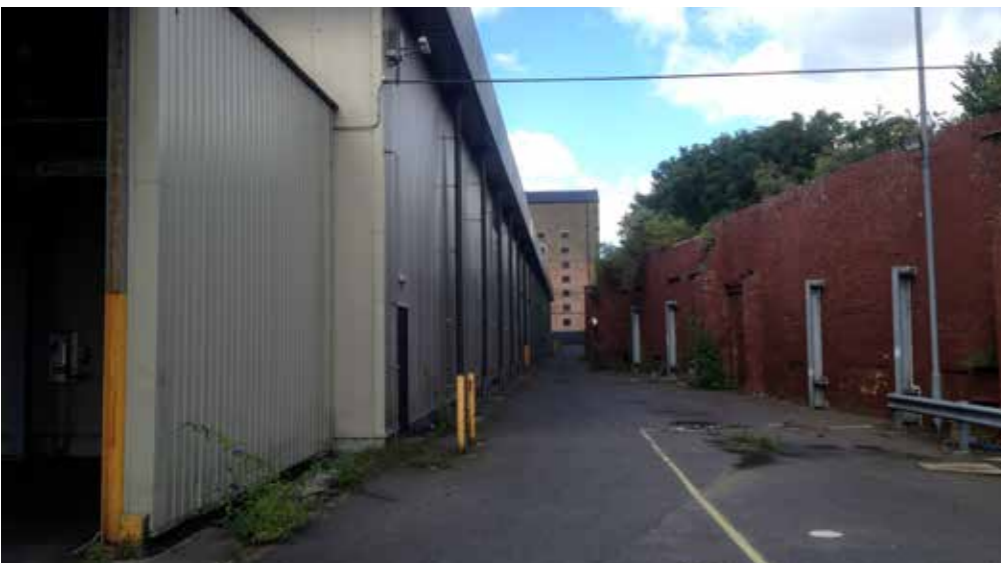
Photo 8 The perimeter wall with the eastern facade of the Maltings at the end
