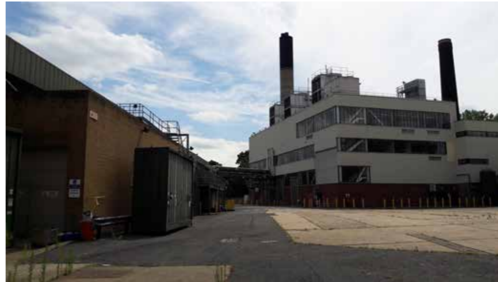
Photo 6 Brewery Buildings to the west of Ship Lane from south
