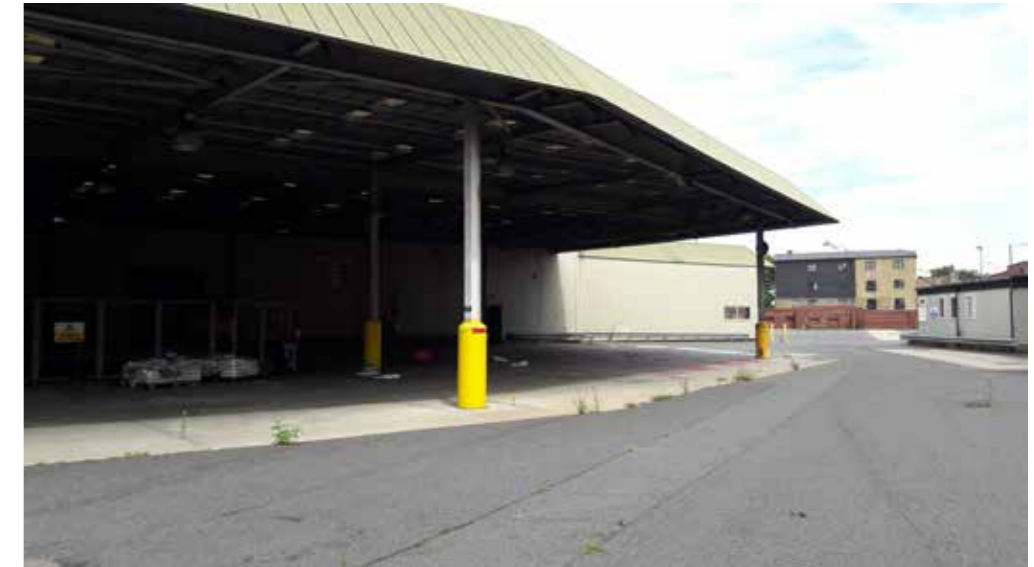
Photo 7 Packaging building to the east of Ship Lane
