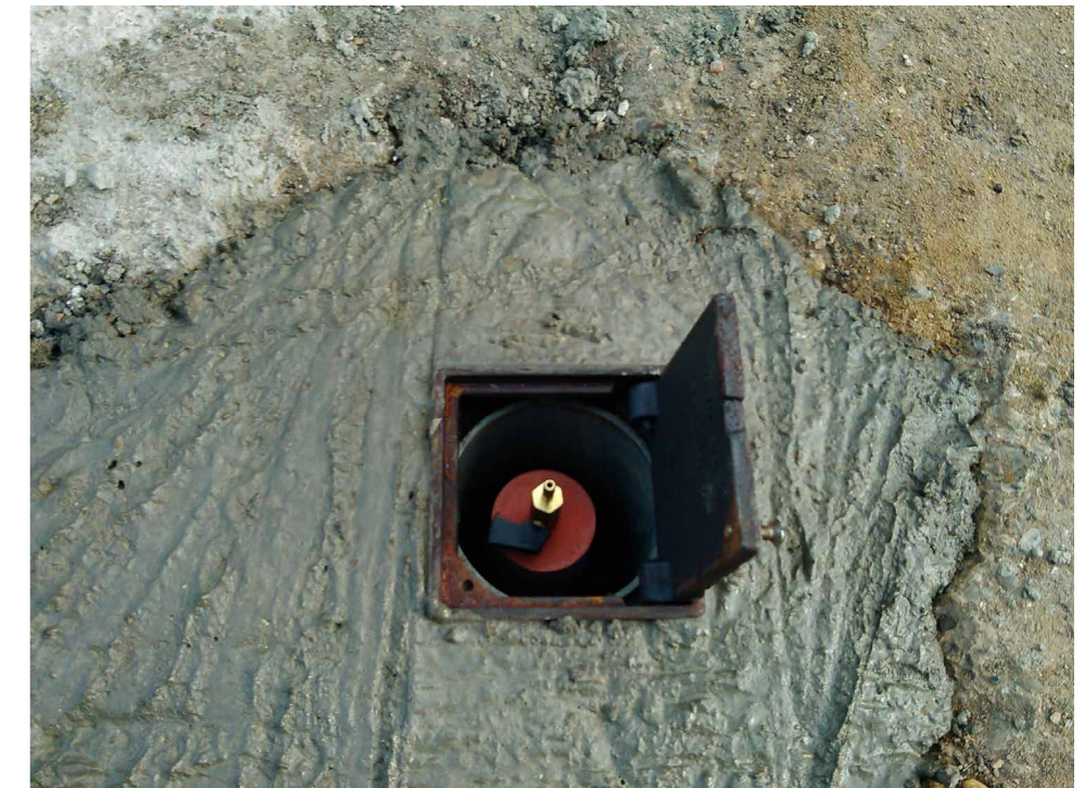
Photograph 8. Typical completed borehole
