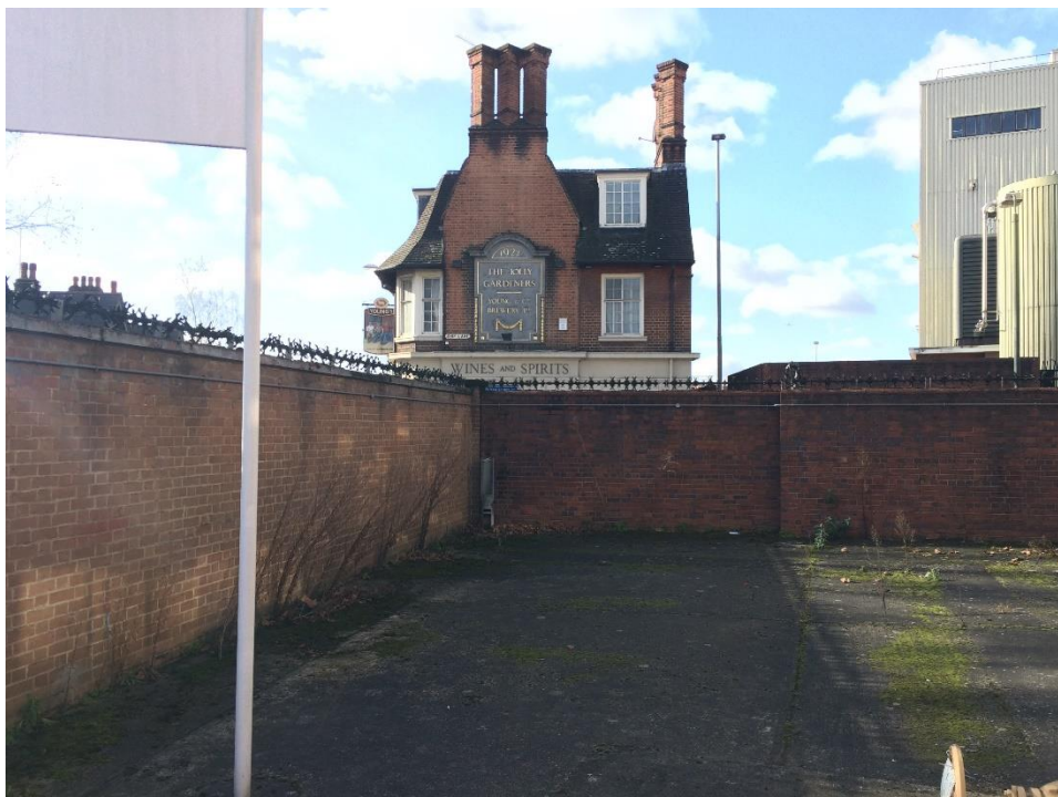
Plate 4 – Brick wall located along the southern boundary of the Stag Brewery component of the Site.
