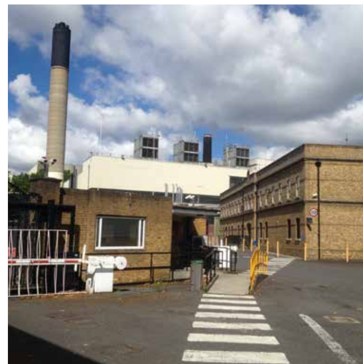
View towards Energy Centre and Packaging Warehouse
