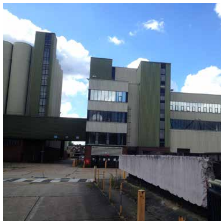
View towards Brewhouses and Finishing Building
