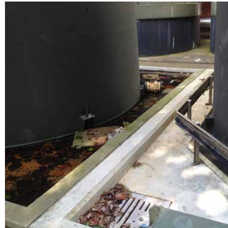
Condition of tank sumps
