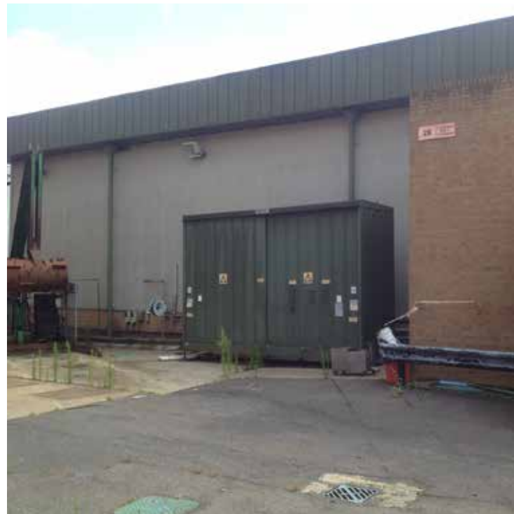
Chemical stores at Packaging Warehouse
