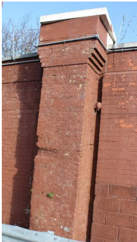
Figure 39: Interior elevation, showing gate pier and surviving hinge socket
