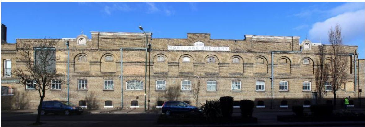
Figure 23: Southern elevation of former Bottling building.
