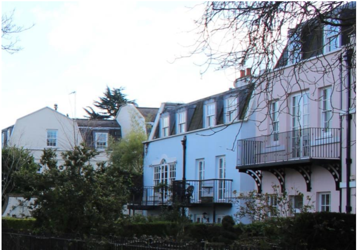
Figure 56: 6 and 7 Thames Bank and corner of Riverside House
