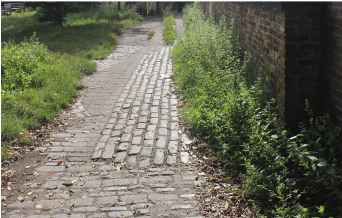
Figure 46: Granite paving setts
