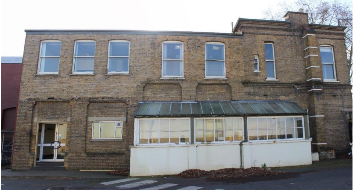
Figure 21: North facing elevation of Former Hotel
