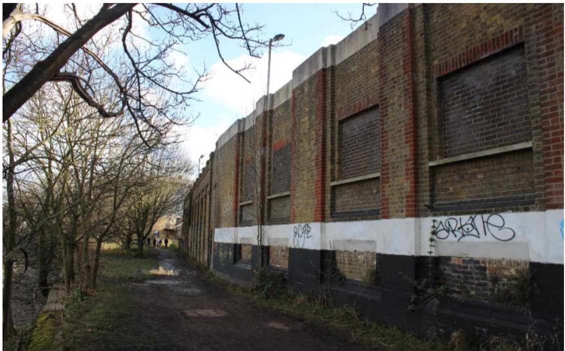
Figure 2: Section 3 - Wall of 1937 Tun Block
