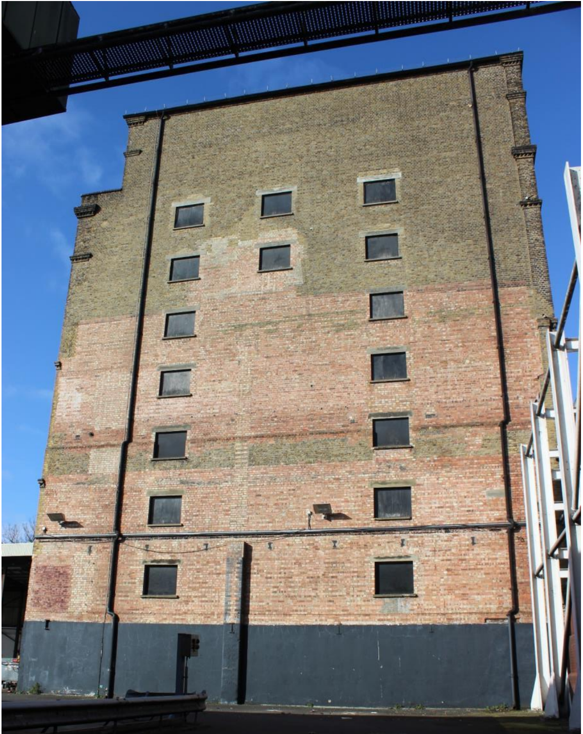
Figure 31: East facing elevation of Maltings
