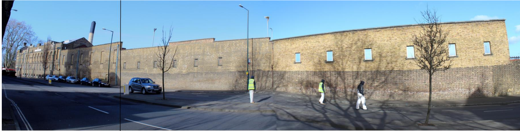
Figure D - Southern Boundary Wall Montage
