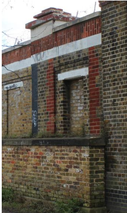
Figure 39: Interior elevation, showing gate pier and surviving hinge socket
