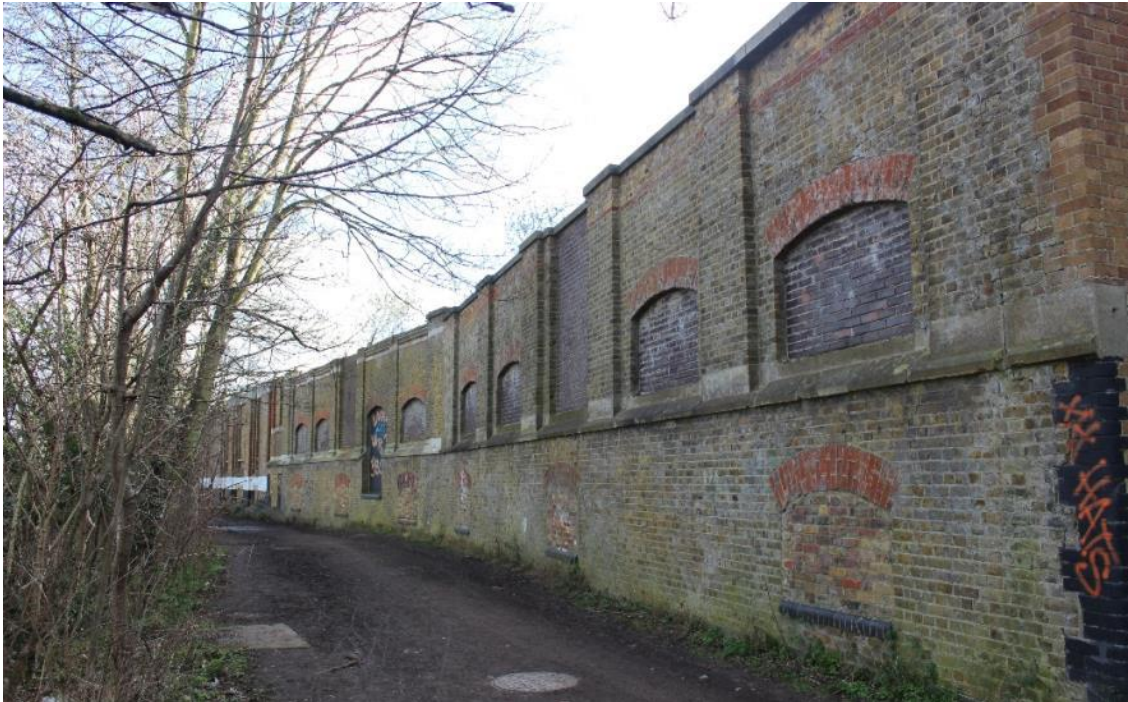
Figure 35: Section 2 - Mid nineteenth century wall
