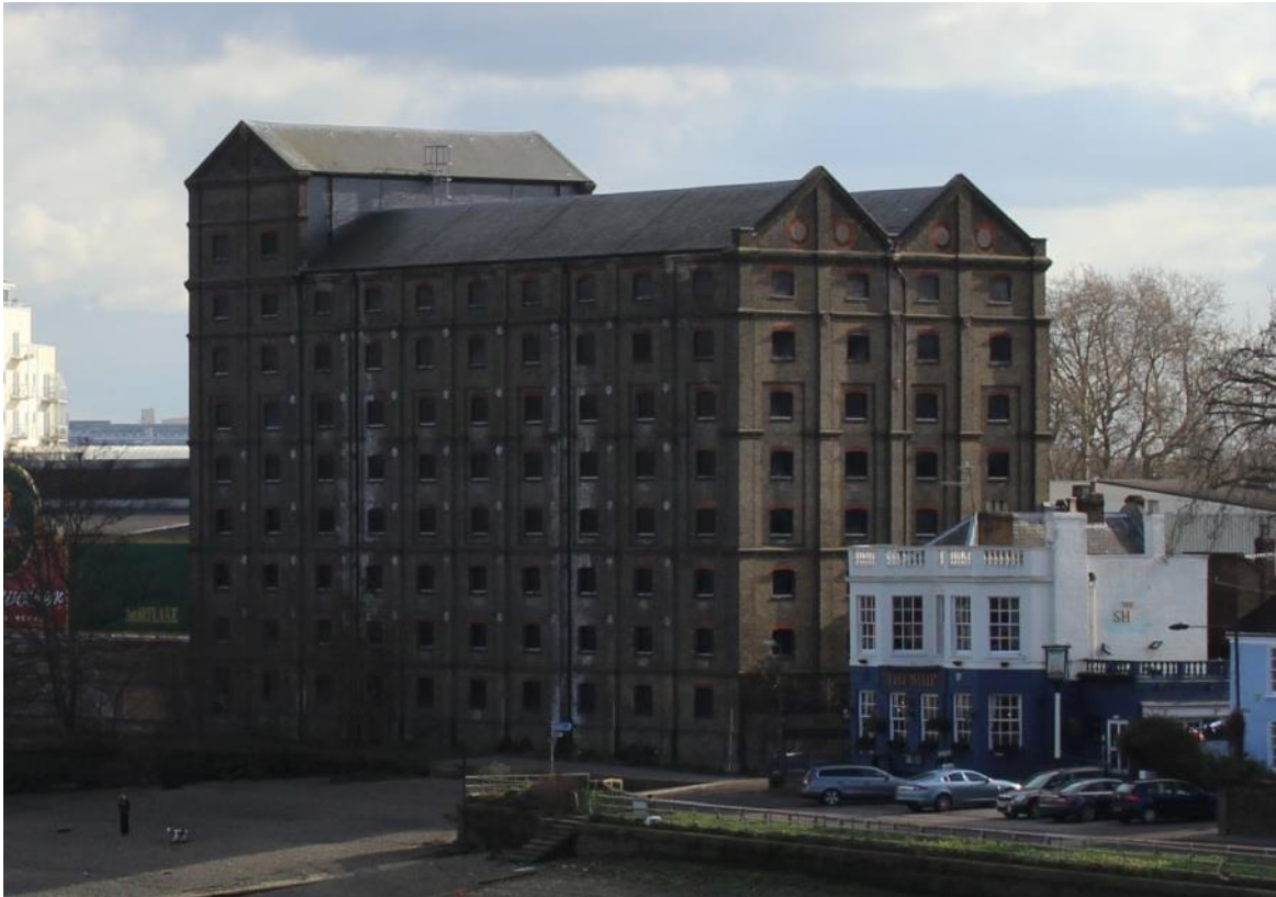
Figure 30: West facing elevation, as seen from Chiswick Bridge
