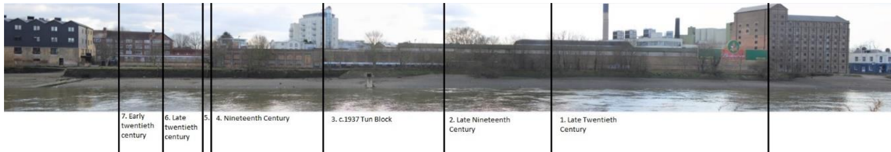
Figure C - Northern Boundary Wall Montage
