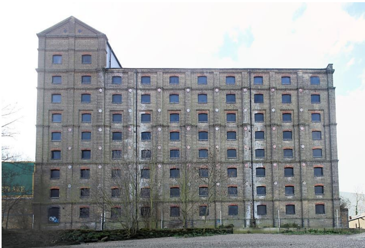
Figure 28: North facing elevation of Maltings.
