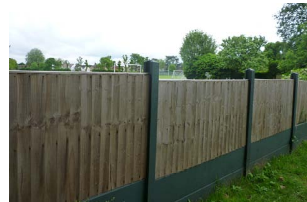
5 - Udney Park Road - Timber panelled boundary wall
