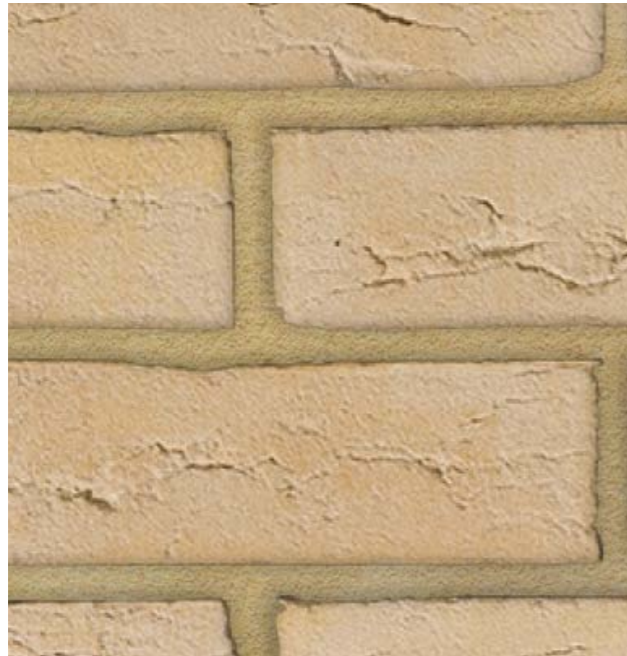
1. Face brickwork with sand colour mortar
