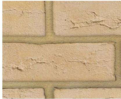
1. Face brickwork with sand colour mortar
