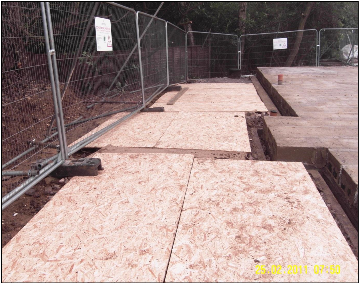
Fig. 1 Ground protection – hoarding over sharp sand and wood chip
