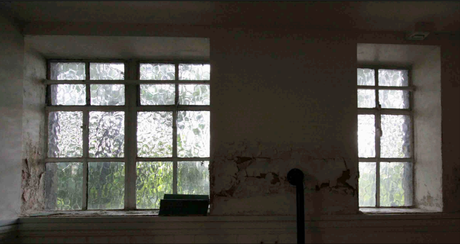
Existing Metal Casement at the Rear inside Showing Decay
