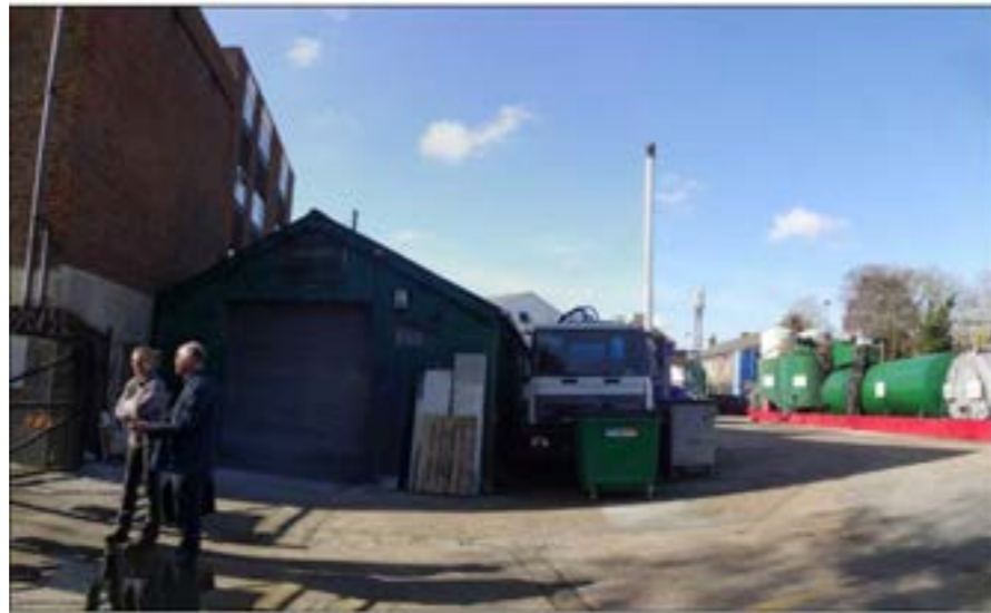
Arlington Works Garages and Recycling Oil Tanks
