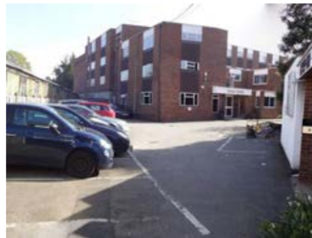
View of Twickenham Studios from Behind Existing Garages
