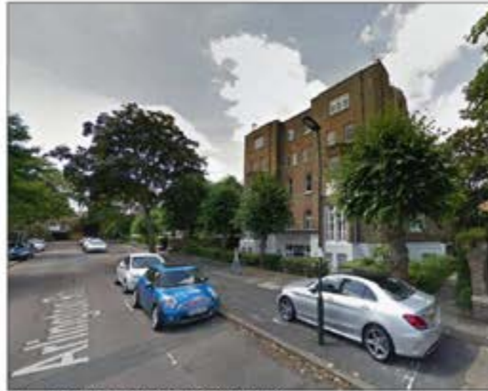
H. Block of Flats on Arlington Road
