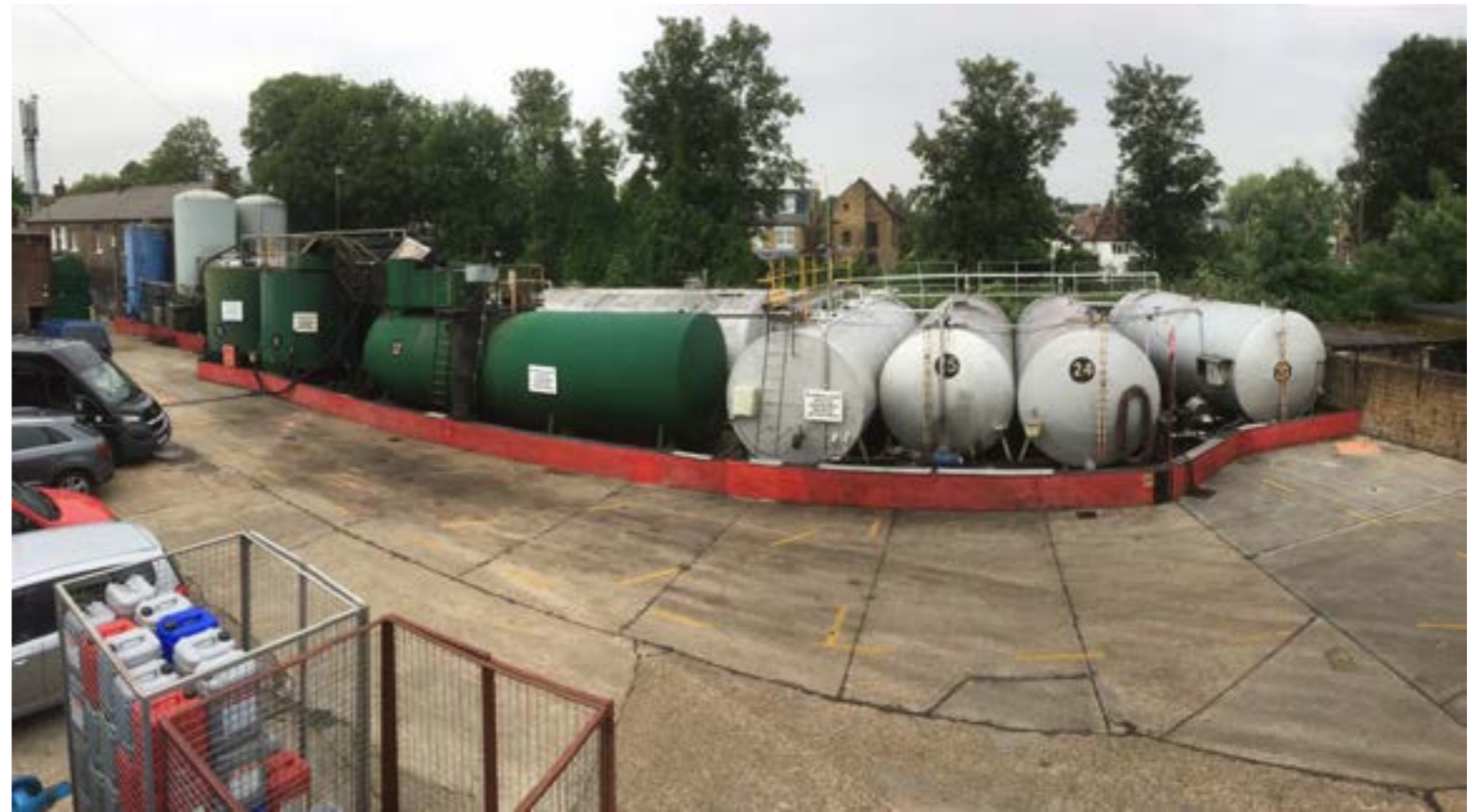
View of Arlington Works Oil Tanks Towards Buildings of Townscape Merit
