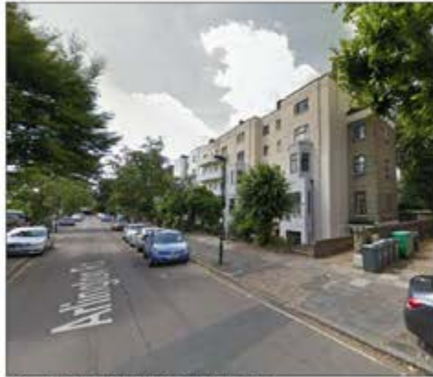
G. Block of Flats on Arlington Road
