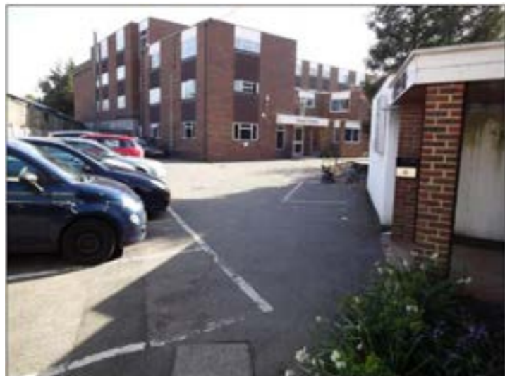
Rear of Arlington Works Garages Looking Towards Twickenham Studios
