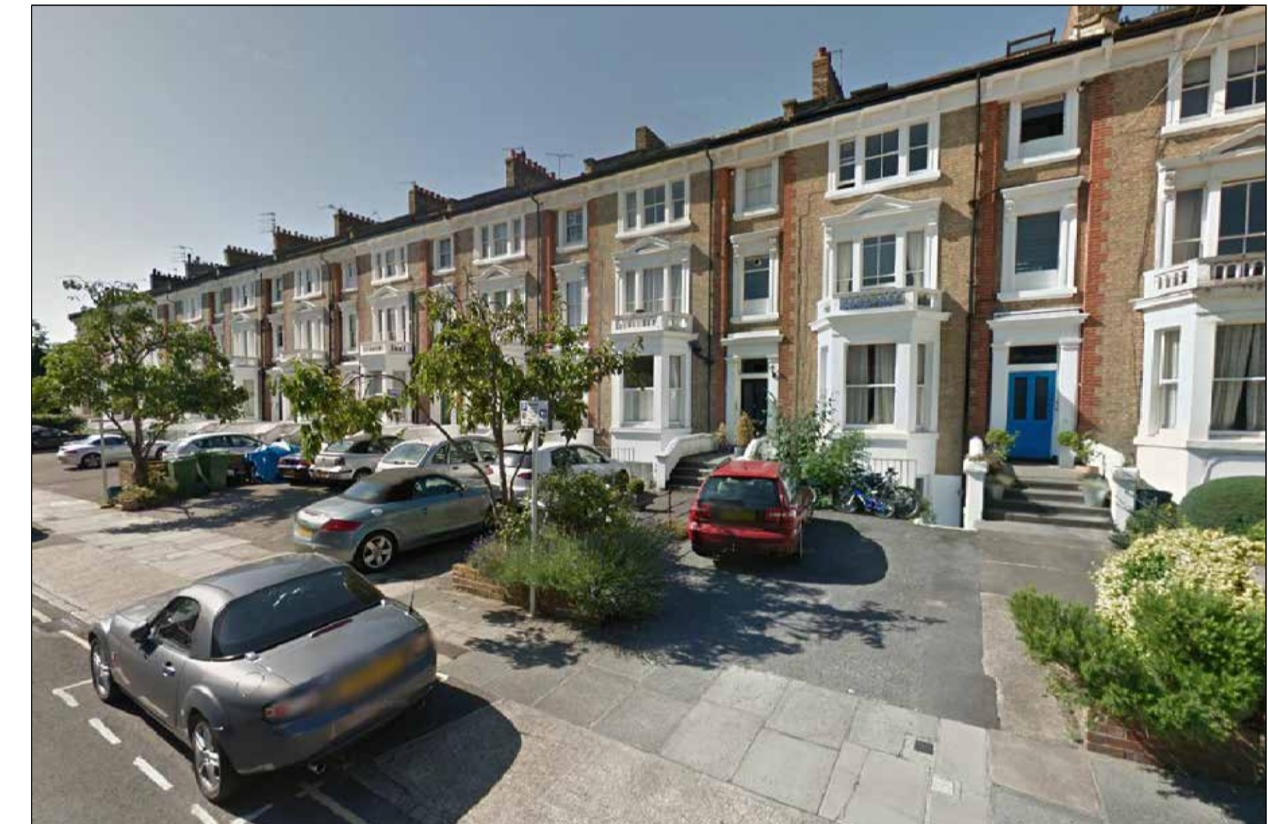
L. Terraced Blocks of flats on Barrons Road
