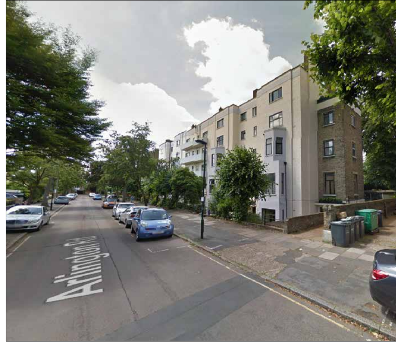
G. Block of flats on Arlington Road
