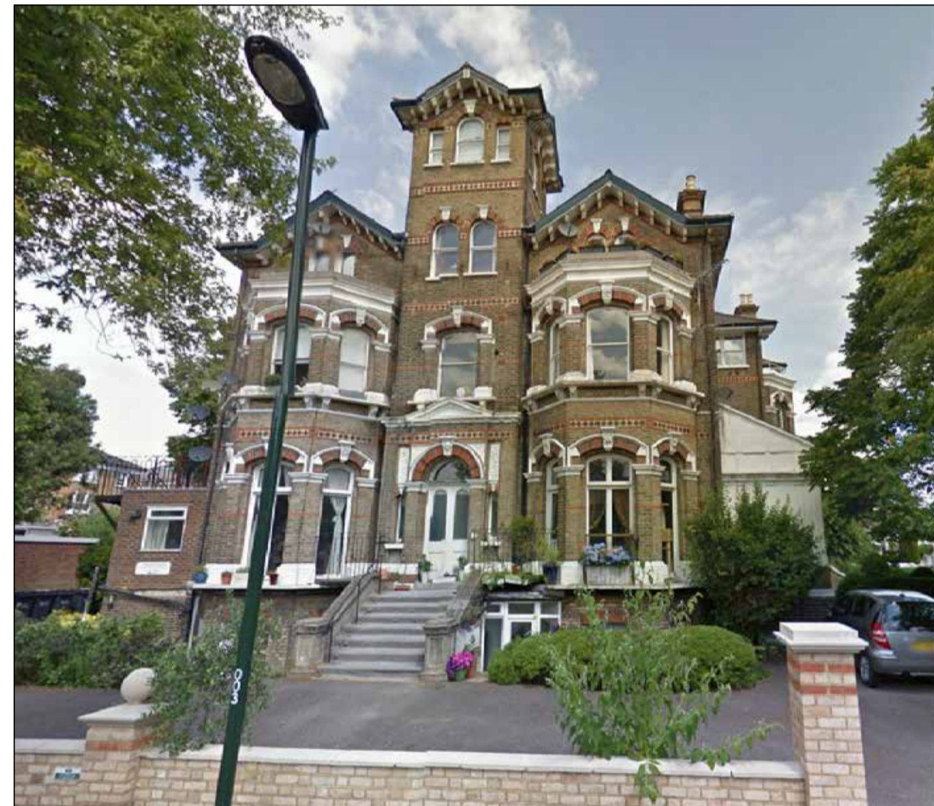
J. Block of flats on Rosslyn Road
