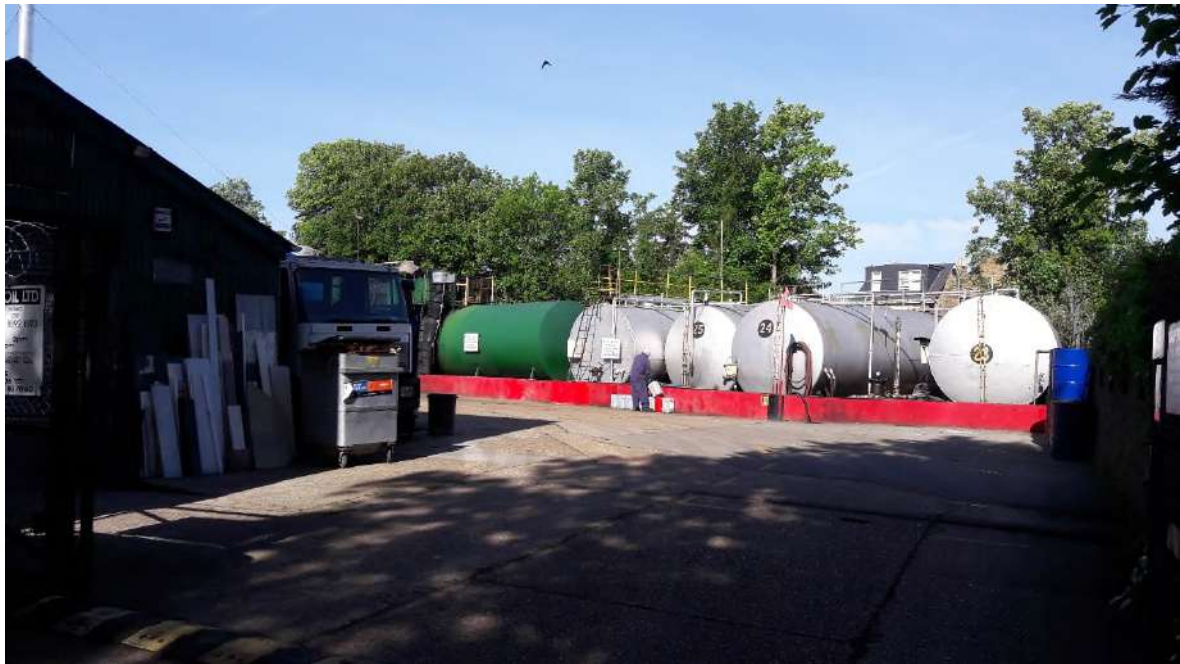
Plate 1: View of the tank farm from the site entrance
